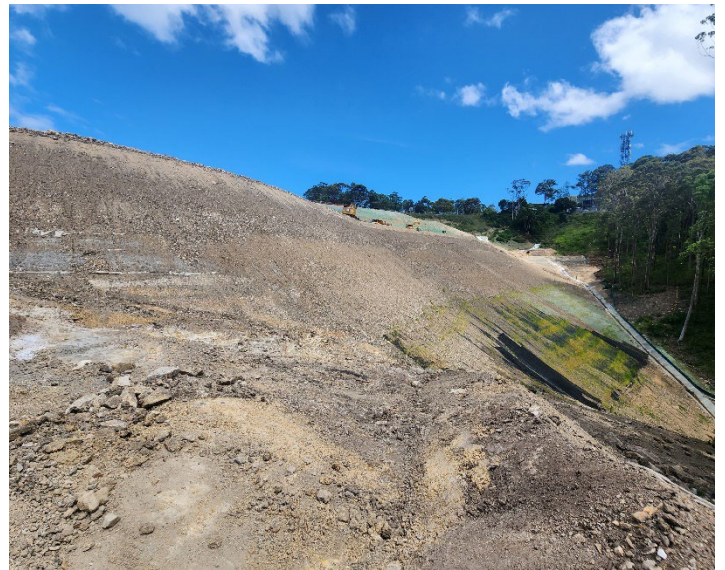
Image 8: Southern Interchange, the batter is in the process of being stabilised with various forms of final landscape designs.
