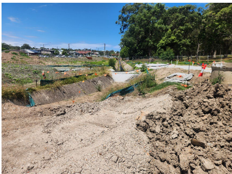
Image 3: Northern Interchange, view of the works on the southern side of Dark Creek. the culvert diversion can be seen in the photo, being used as a temporary sediment basin.
