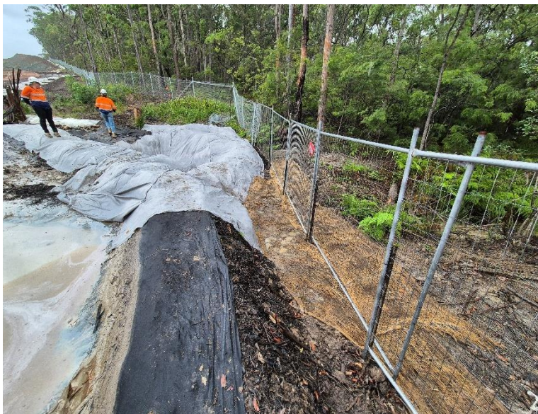
Image 7: Mainline near Creek 3 showing repairs to ErSed controls and remediation of surrounding area following major rain event.
