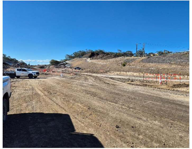
Image 6: View looking south along the mainline. shotcrete carbonaceous batter can be seen in the background and the clean water shotcrete drain the foreground.
