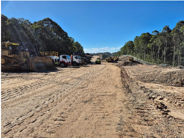
Image 5: View looking north along the mainline. The finished road height has almost been reached.
