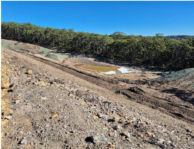
Image 7: Mainline near Creek 3 showing sediment basin and clean water drain on the western side of the corridor.
