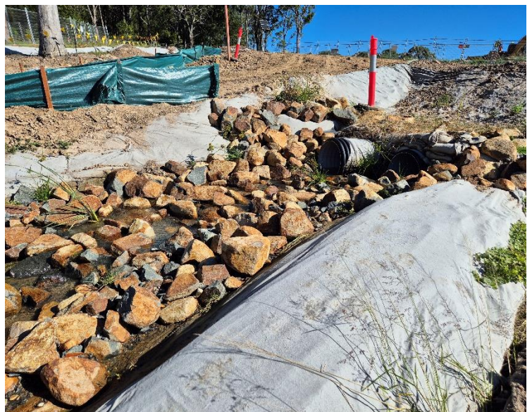
Image 4: Clean water drains at the Northern Interchange on the Southern side of Newcastle Road.
