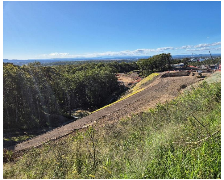
Image 8: View of the Southern Interchange looking north from Lookout Road. The light green on the batter is recent revegetation using MacMat and hydromulch, which has held up well during the April storms.
