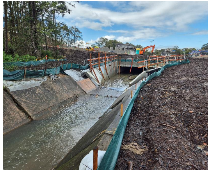
Image 8: Image 7: ErSed controls around Zone 1, which drains into Dark Creek (concrete culvert). View looking south (upstream)
