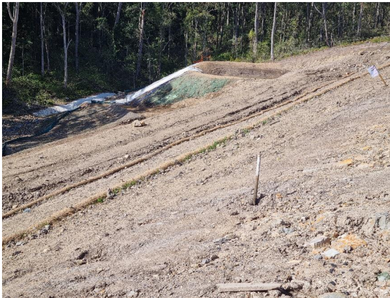
Image 7: View sediment basin at the southern end of the mainline following desilting and re-establishment.
