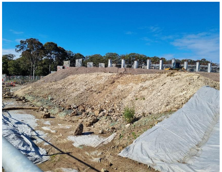
Image 4: Northern Interchange, embankment works for the southern side of the Newcastle Road overpass.
