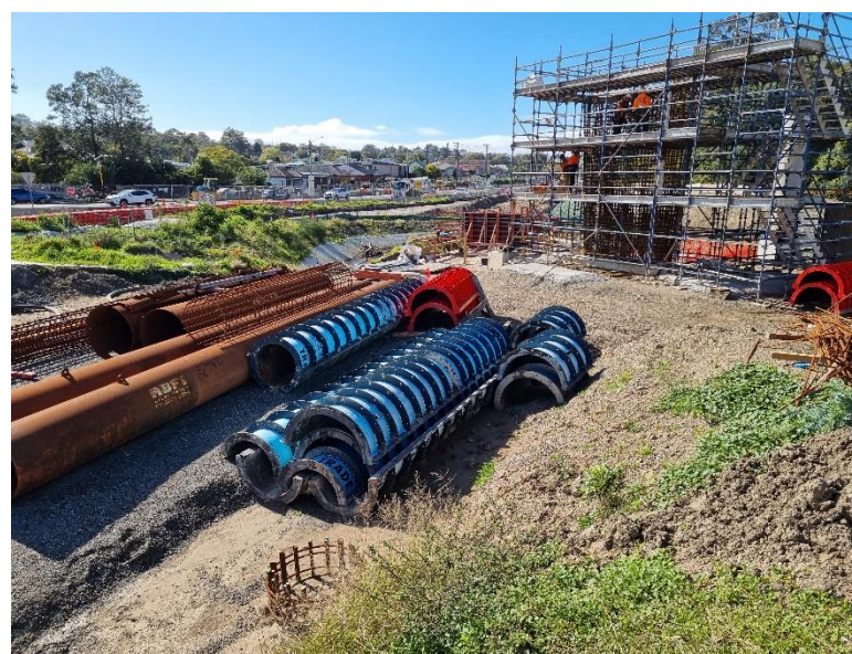
Image 1: Northern Interchange, photo is taken of the formwork for the bridge footings for the onramp.
