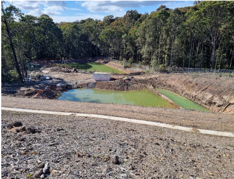
Image 5: Mainline, inspection of eastern sediment basin and water storage basin.
