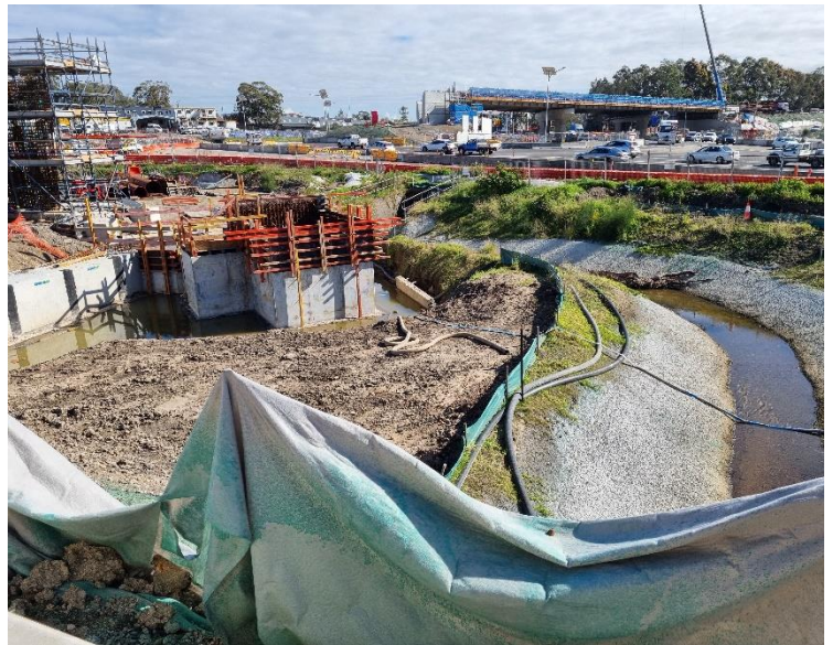
Image 2: Northern Interchange, photo is taken of the dark creek temporary diversion and construction of the Dark Creek culvert.
