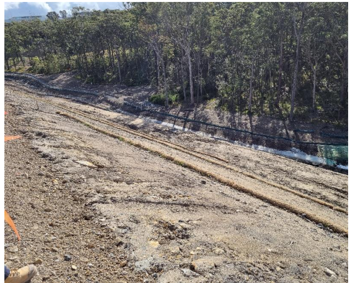
Image 8: Mainline, view of the ErSed controls and permanent landscaping works on the eastern boundary below the JHH car park.
