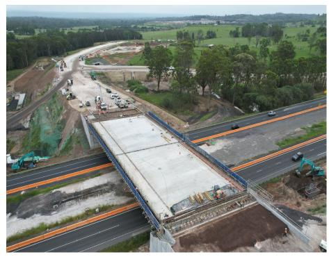
Work is continuing to advance on Spring Farm Parkway Stage 1. Since our last update, we have built several key features of the east to west bridge link over the Hume Motorway. This work has included pouring of the concrete deck and installing the bridge safety barriers.
