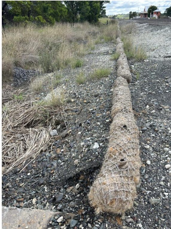
Photo 7: Middle culvert upgradient of the railway line with no flowing surface water. Minor observed build-up of sediment on rocks.
