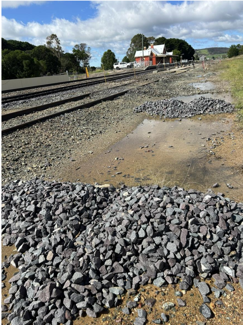
Photo 14: Rock checks and rock armour appeared in good condition.
