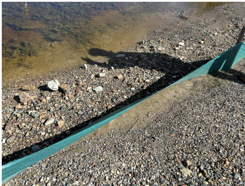
Photo 8: Middle culvert upgradient of the railway line with no flowing surface water. Observed build-up of sediment fencing.
