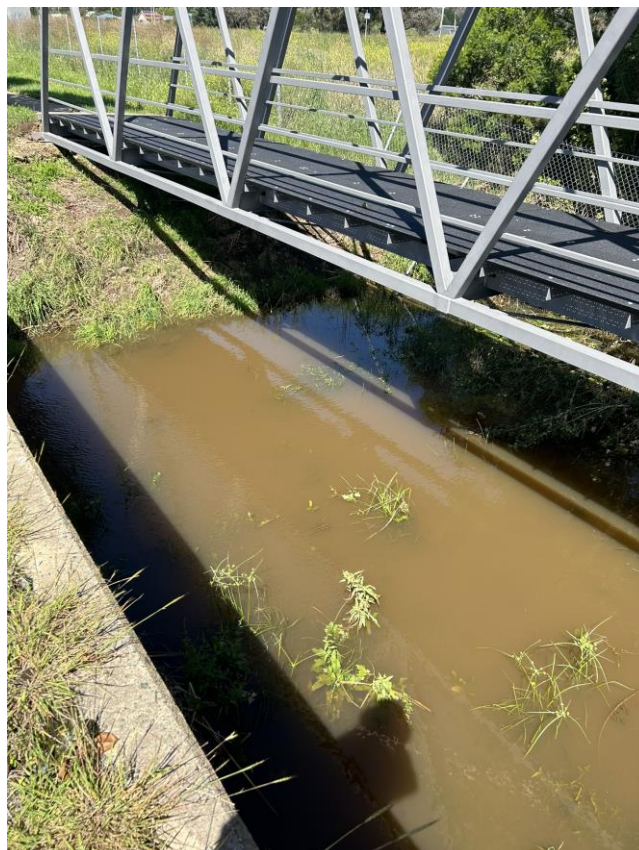
Photo 10: Water flowing out downgradient of the site, light brown and turbid.
