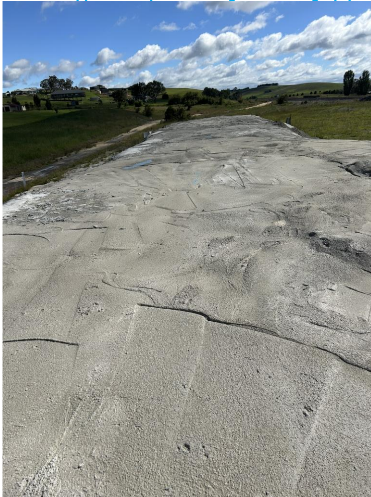
Photo 14: Concrete capped stockpile. Top surface, undamaged, no sign of cracks.
