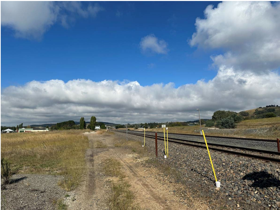
Photo 2: Picture of Tarago railway facing south west towards platform. No airborne dust visible.
