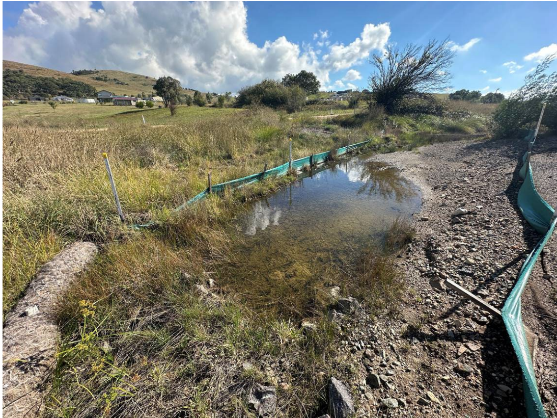
Photo 15: Upgradient of middle culvert. Pooled surface water on site was clear with no turbidity. Sediment controls in place (coir logs and rock armoury in average condition).
