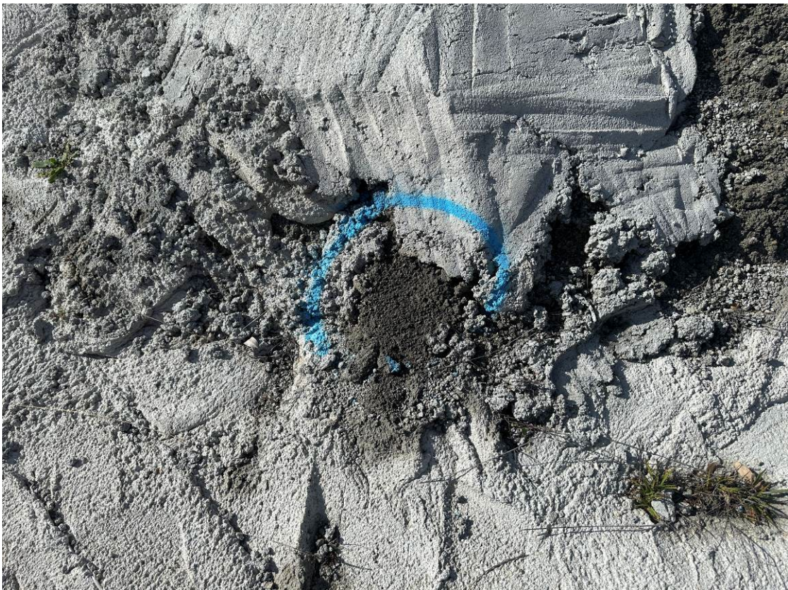
Photo 18: Previously exposed geofabric layer marker on stockpile, noted during March EMP Inspection had been filled with cement.
