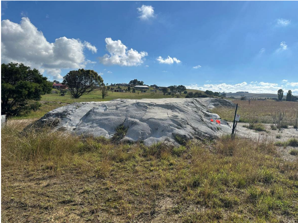
Photo 19: Concrete capped stockpile. No major signs of exposure marker layer and erosion damage. Some vegetation growing but not expected to impact capping integrity.
