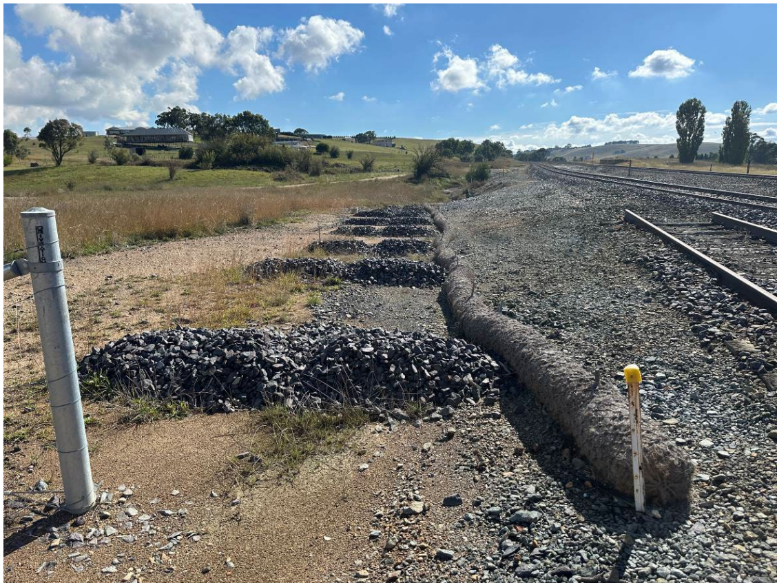
Photo 13: Upgradient of middle culvert. Sediment controls in place (coir logs and rock armoury in good condition).
