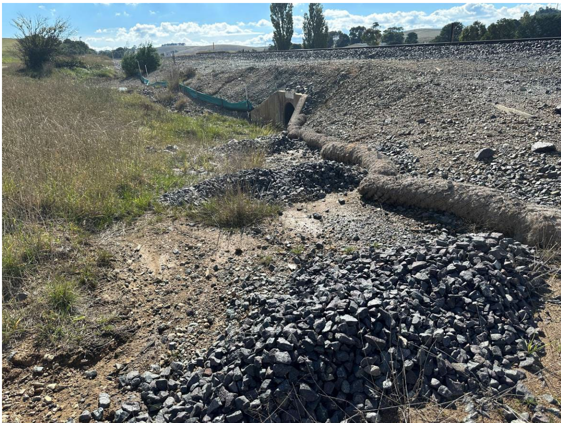
Photo 14: Upgradient of middle culvert. Sediment controls in place (coir logs and rock armoury in good condition).
