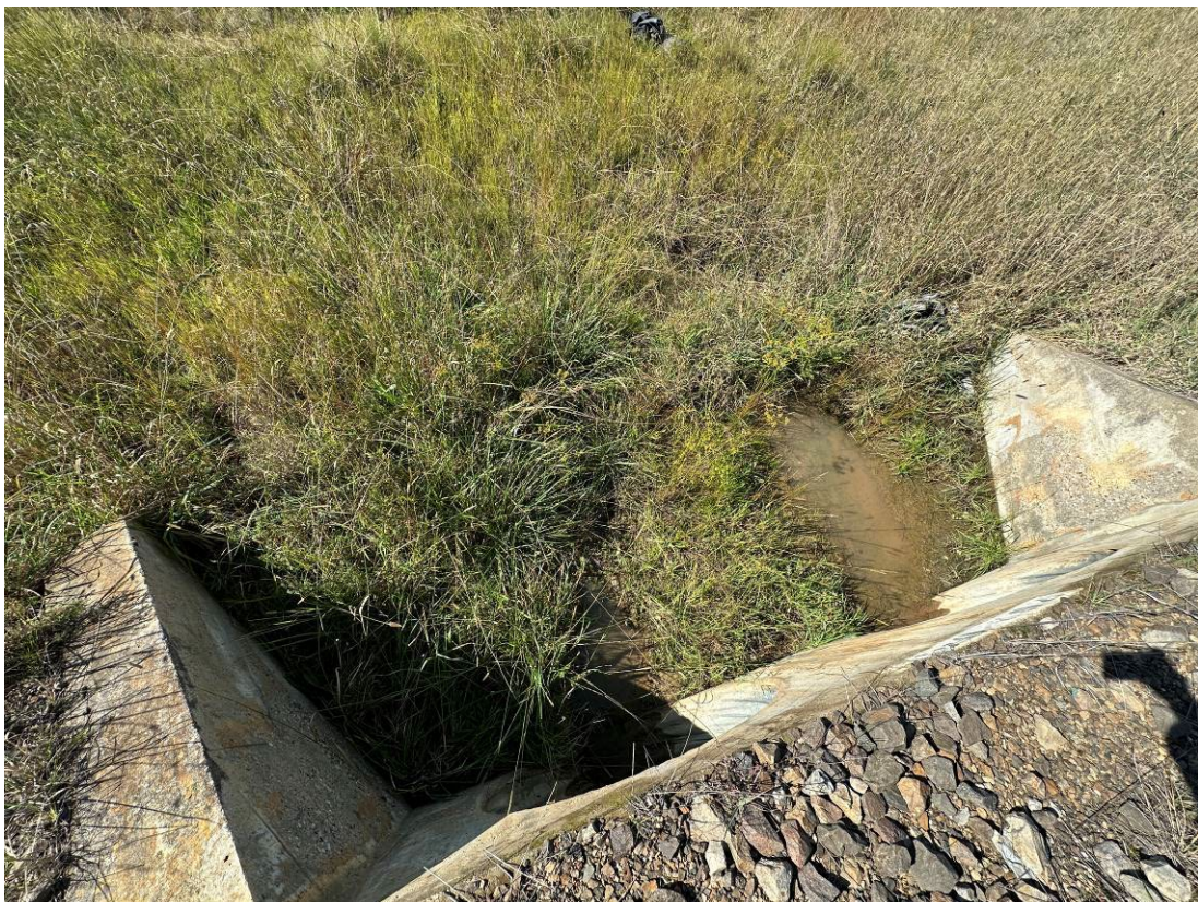
Photo 8: Downgradient of northernmost culvert with pooled surface water. Water was clear with slight brown tint, and low turbidity.
