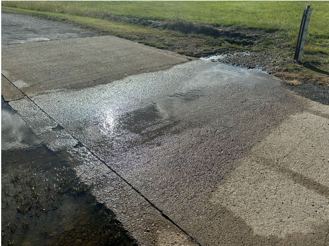
Photo 7: Causeway located downgradient of middle culvert facing east with pooled surface water. No sediment located on causeway.
