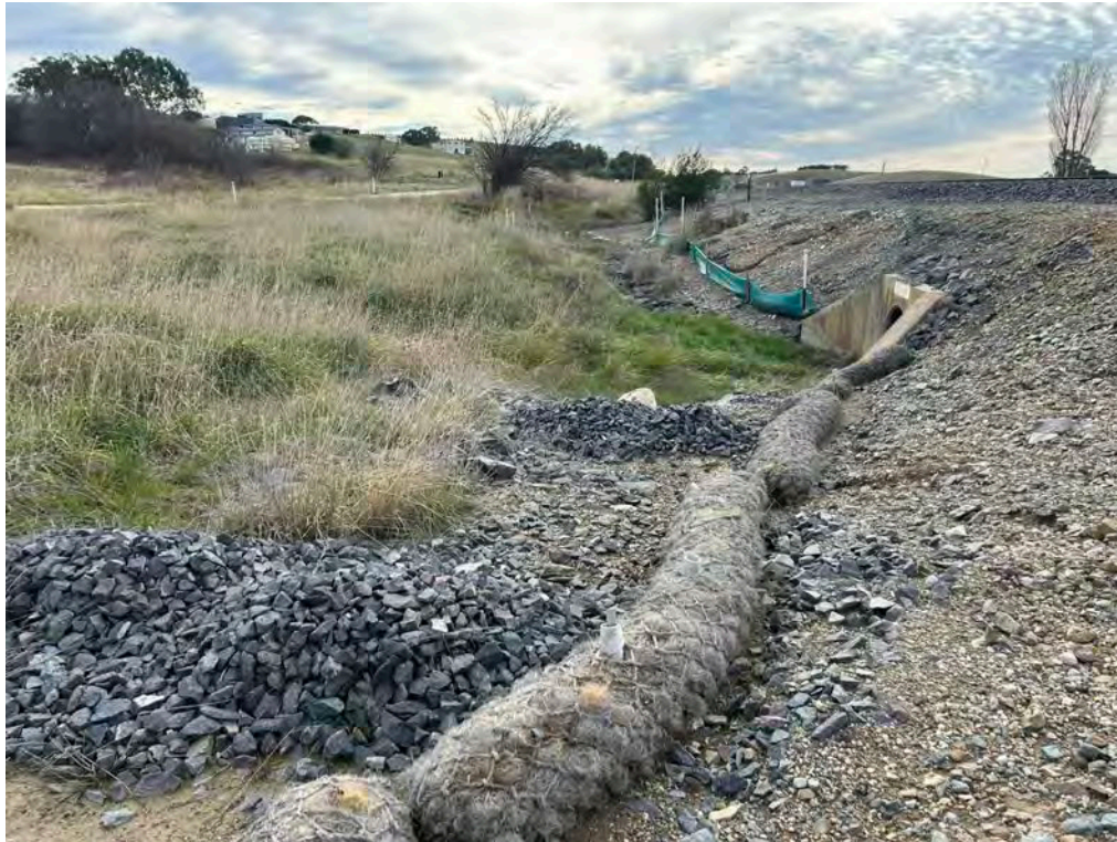
Photo 11: Rock armoury and sediment coir logs following drainage to upgradient of middle culvert in good condition with minor build-up of sediment
