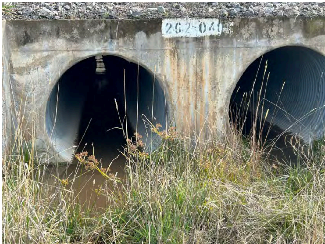
Photo 6: Downgradient of northernmost culvert with pooled surface water. Water was moderately turbid with slight brown to grey in colour. Not flowing off site to adjacent property.
