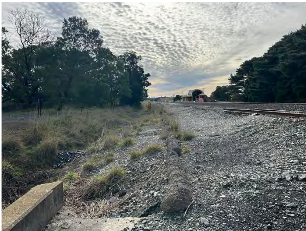
Photo 8: Southernmost culvert upgradient of the railway line. Sediment control coir logs in place and in good condition.
