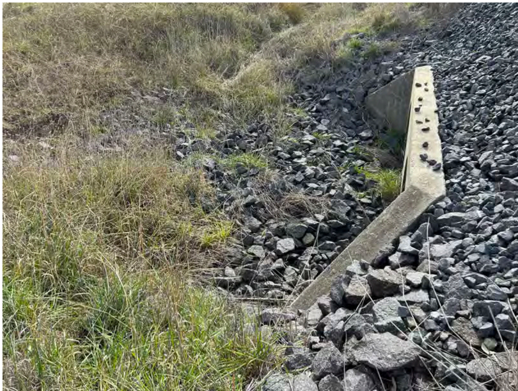
Photo 15: Upgradient of northernmost culvert with no surface water. No sediment build up was noted on rock armoury.
