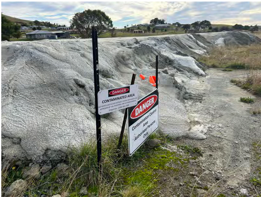
Photo 16: The concrete-capped stockpile is in good condition with no evidence of erosion. One contamination sign on the southeastern corner was slightly damaged but fixed by UGL personnel on site. All other signs were intact and in good condition.
