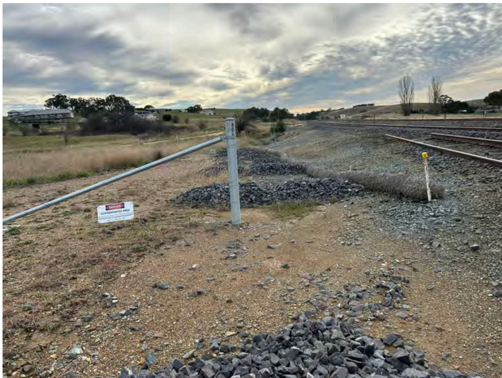
Photo 10: Rock armoury and sediment coir logs adjacent to old rail siding in good condition. No surface water was observed.
