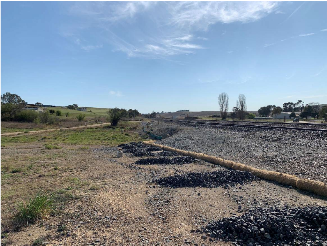
Photo 12: Rock checks running alongside former Woodlawn siding towards the middle culvert. No evidence of sediment build-up in rock armoury or Coir sediment control logs.
