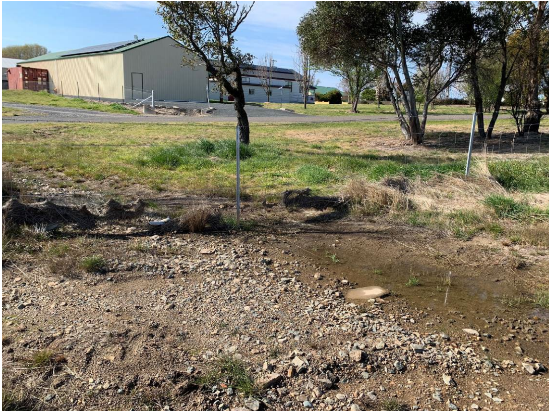
Photo 19. Downgradient of middle culvert. Water is pooled adjacent to site boundary fencing. Extending to off-site damp soil, in line with the pooled water, was visible suggesting former run-off. No current water running off from site.
