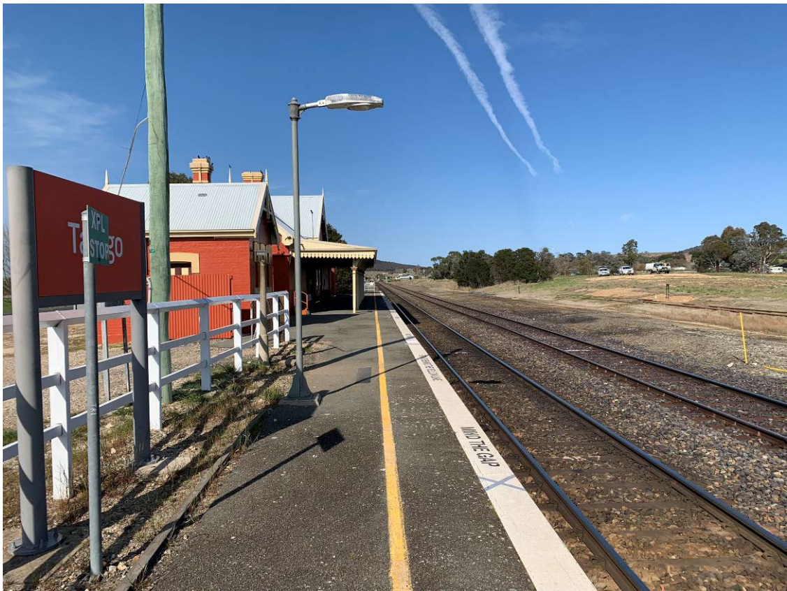
Photo 1: Picture at north-east end of railway station facing south-west. No airborne dust visible.
