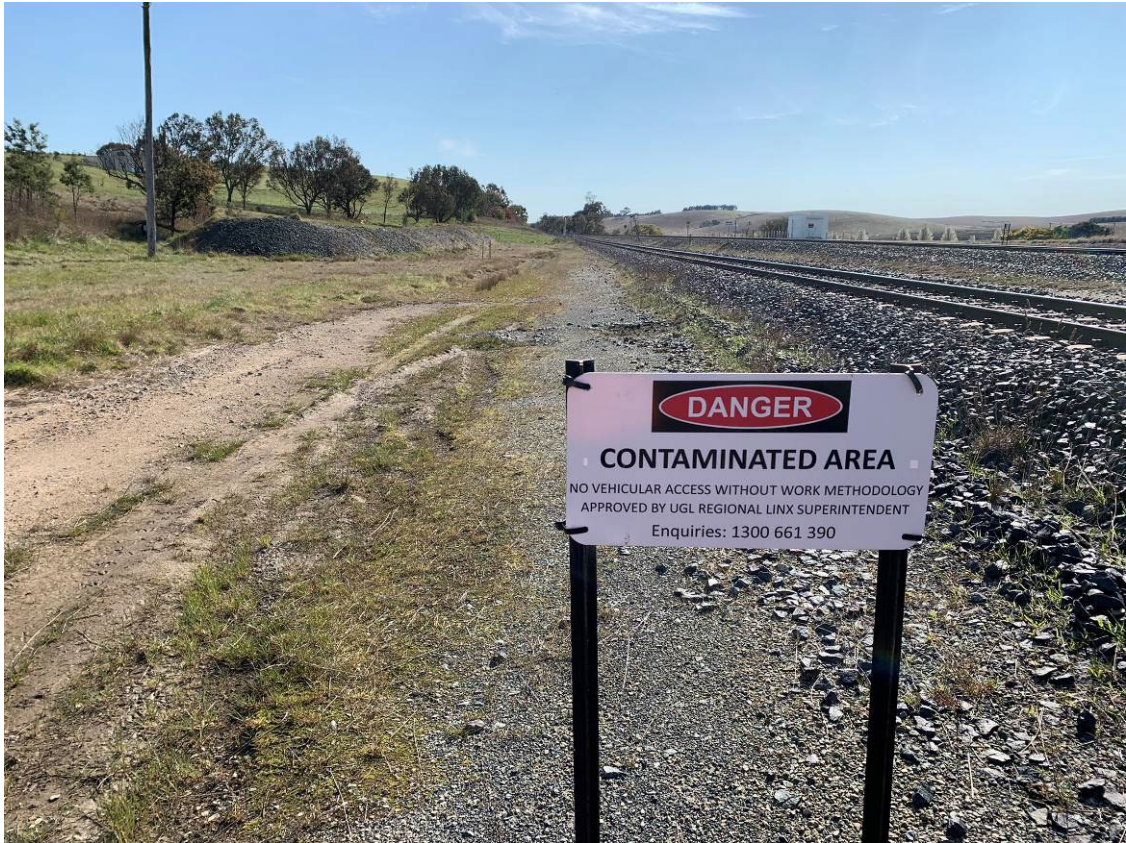
Photo 17: Exclusion zone signing placed periodically along contamination areas. Undamaged and in good condition. Facing North-East.
