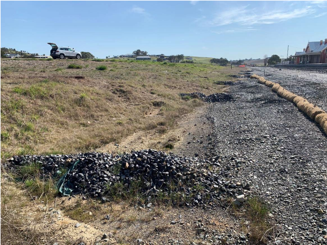
Photo 11: Rock checks running along former Woodlawn siding and between southern and middle culverts. Silt fencing replaced by Coir sediment control logs.
