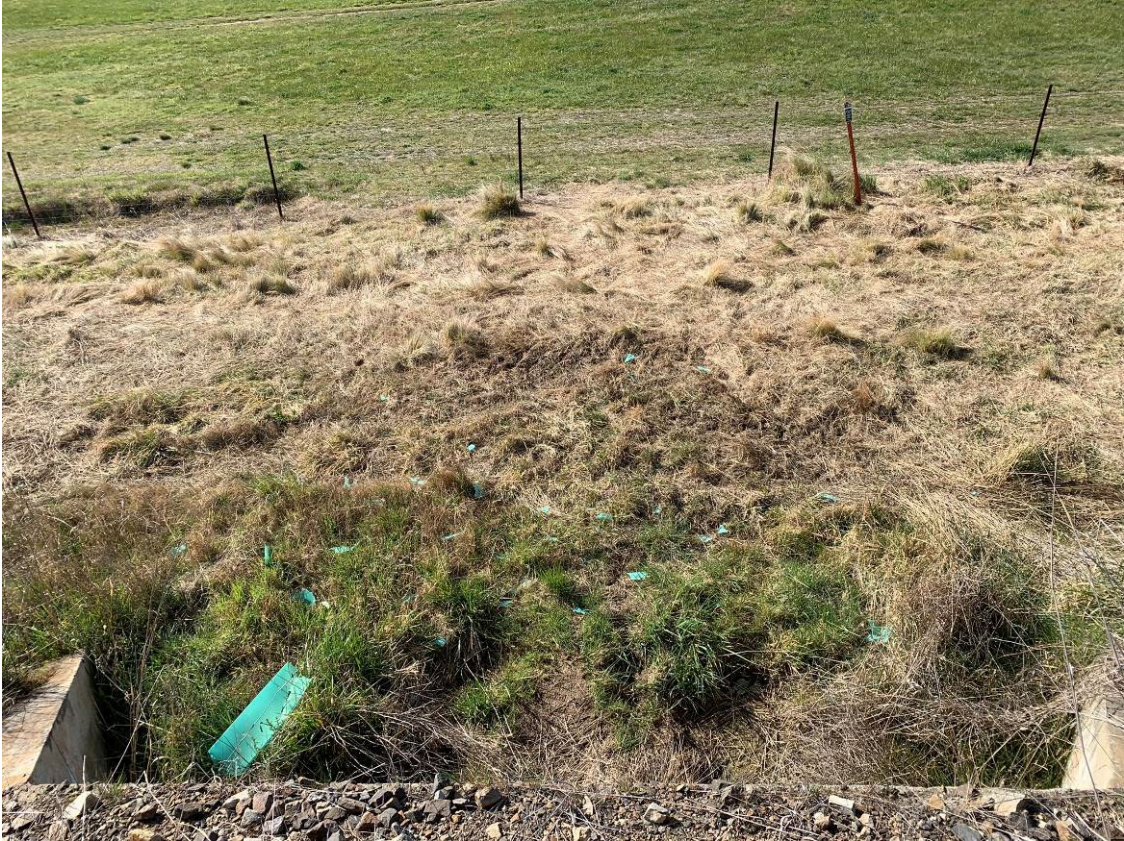
Photo 7: Downgradient of northernmost culvert showing evidence of no surface water runoff from site to neighbouring property.
