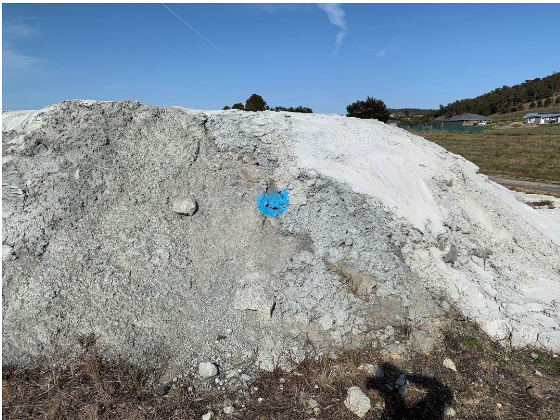
Photo 20: Exposed geofabric layer marker on main stockpile newly identified during the inspection. Marked with blue paint. Facing the south-western side of stockpile.
