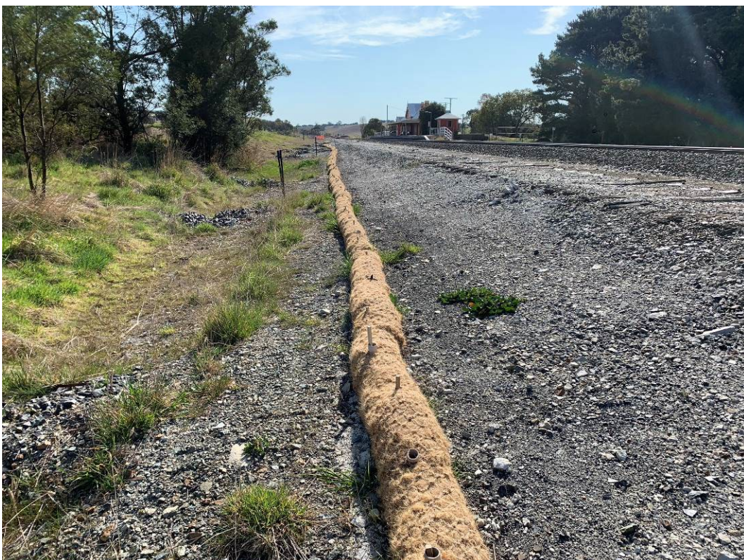
Photo 10: Upgradient of southernmost culvert showing Coir sediment control logs, used as control measures for sediment control. Facing north-east.
