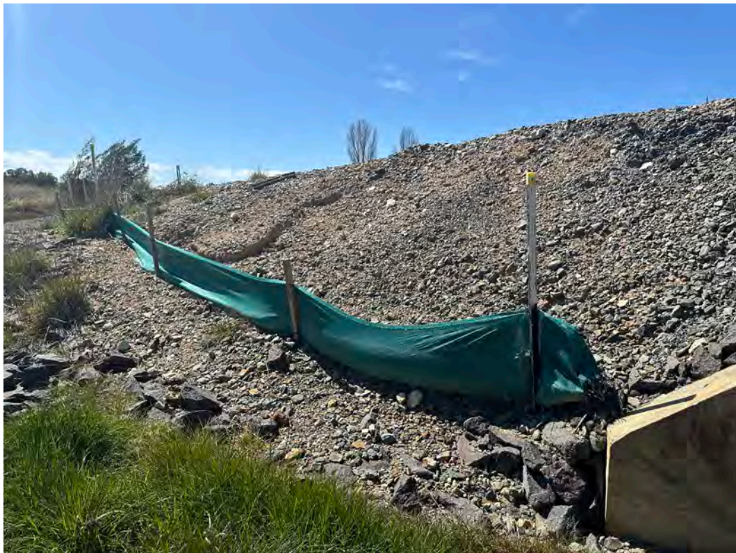
Photo 11: Upgradient of railway line to the north of the middle culvert. Sediment fencing in place with large build-up of sediment. Some minor erosion due to inadequate ground cover was observed.
