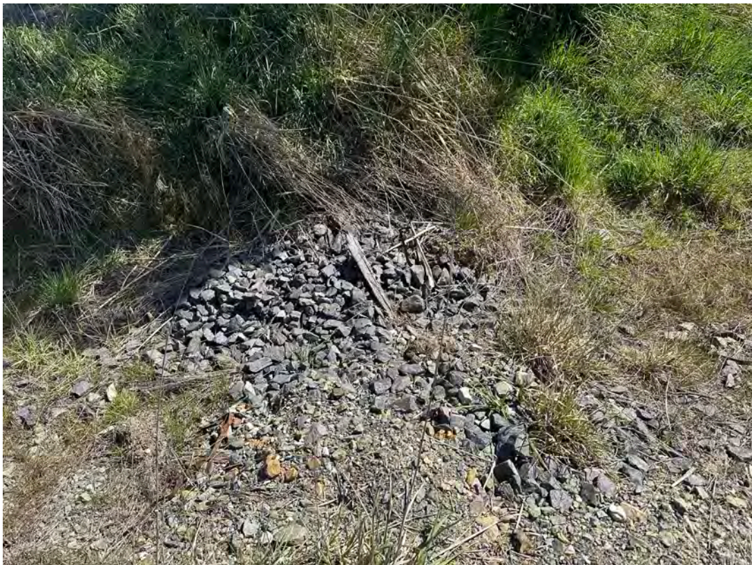
Photo 9: Rock armoury in drainage channel between southern and middle culverts appear to be in average condition, with minor build-up of vegetation and sediment.
