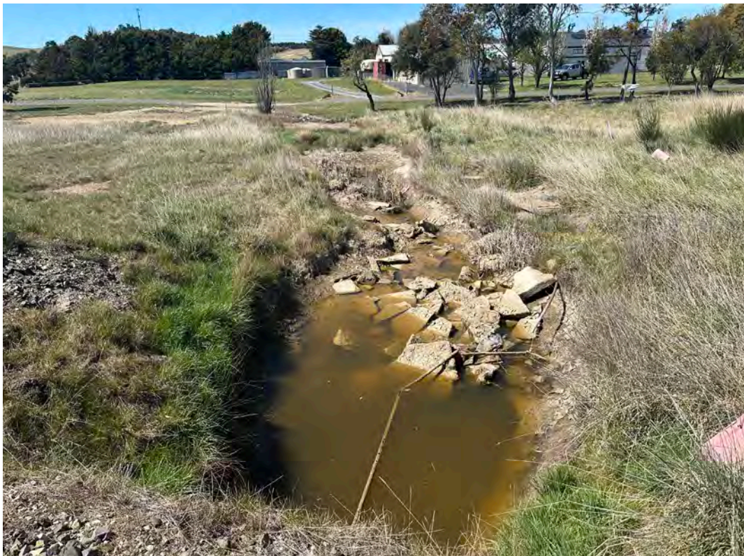
Photo 4: Downgradient of middle culvert with pooled surface water, not flowing off site. Surface water near culvert was slightly brown with minor visible turbidity and suspended solids.
