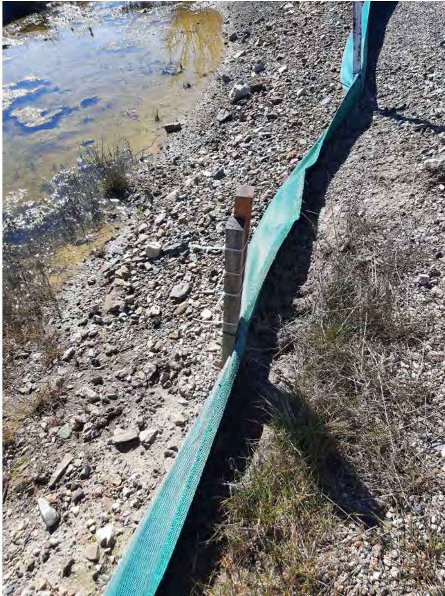
Photo 19: Damage to sediment fencing in drainage line north of middle culvert had been repaired by UGL staff. (Photo provided by UGL).
