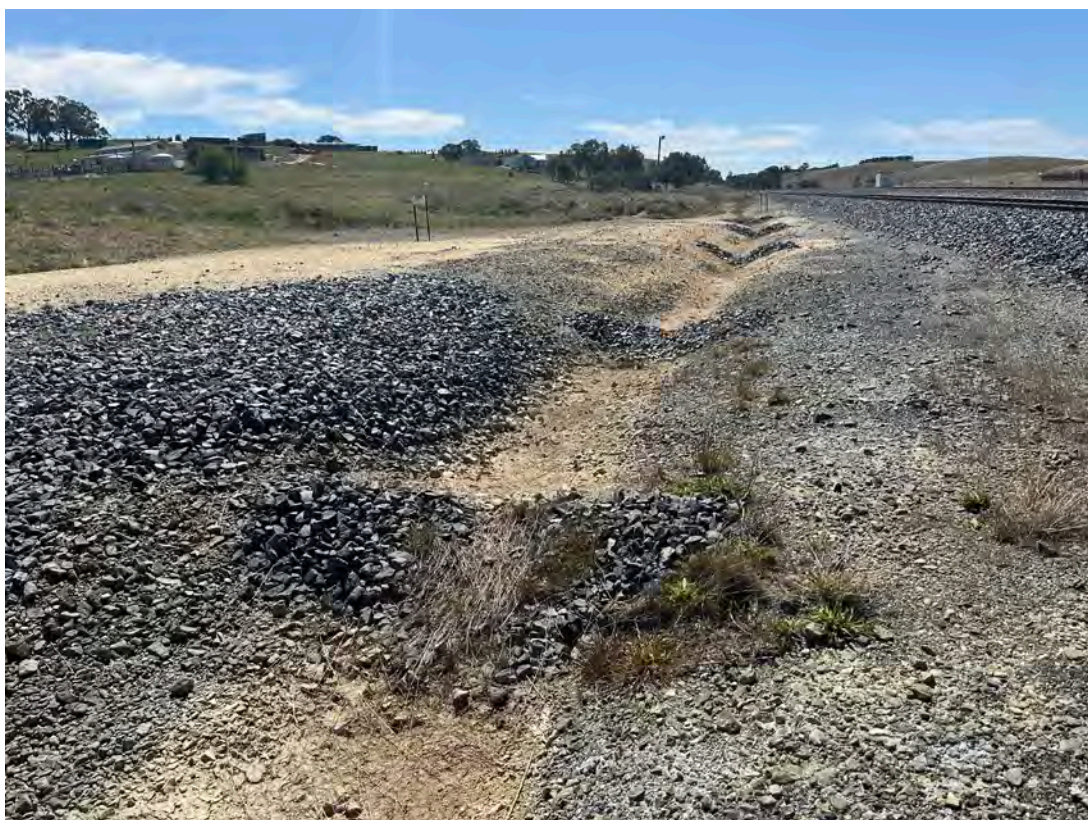
Photo 14: Rock armoury in drainage channel between middle and northern culverts appear to be in good condition with minor vegetation and sediment build up.
