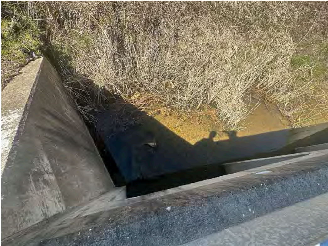
Photo 3: Southern culvert downgradient of railway line with surface water flowing offsite. Surface water was clear with no visible turbidity or suspended solids.
