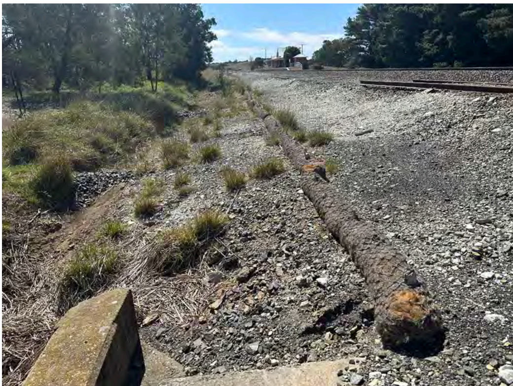
Photo 8: Southernmost culvert upgradient of the railway line. Sediment control coir logs in place and in good condition. Rock armoury in drainage channel between southern and middle culverts appear to be in average condition, with minor build-up of vegetation and sediment.
