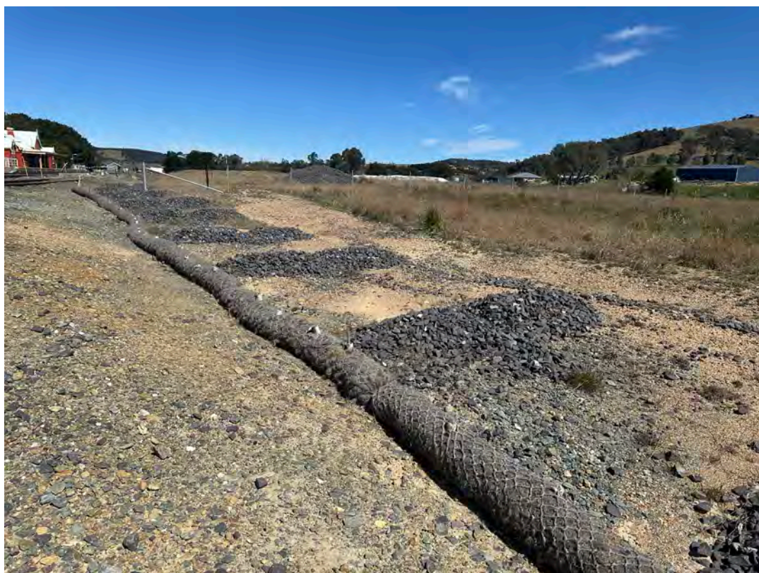
Photo 10: Rock armoury in drainage channel between southern and middle culverts appear to be in good condition, with minor build up of vegetation and sediment.
