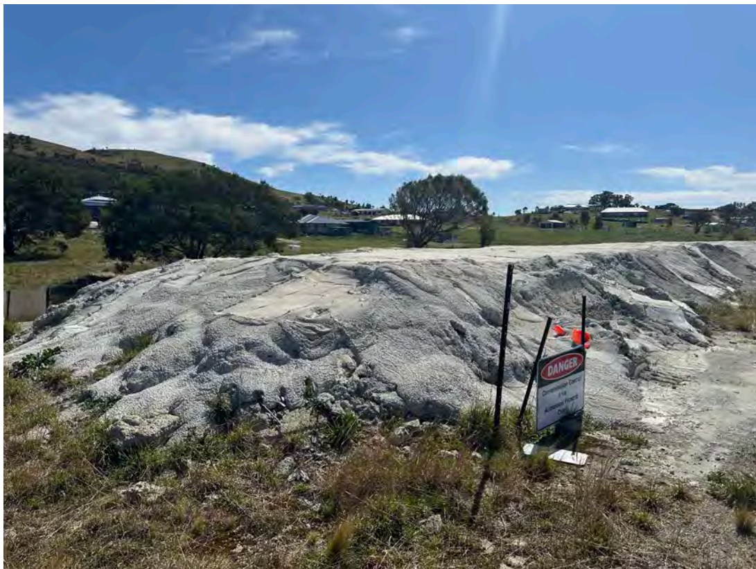
Photo 16: The concrete-capped stockpile is in good condition with no evidence of erosion.
