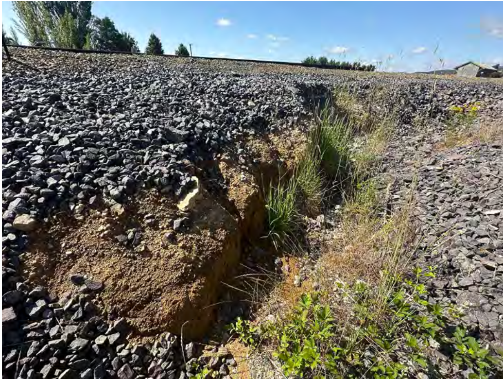
Photo 9: Southernmost culvert upgradient of the railway line. The erosion due to lack of ground cover observed during multiple previous inspections is still present. More vegetation present.
