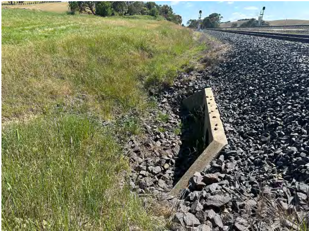
Photo 16: Upgradient of northernmost culvert with no surface water. No sediment build up was noted on rock armoury.
