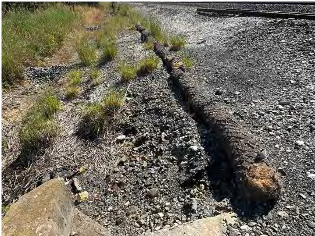
Photo 10: Southernmost culvert upgradient of the railway line. Rock armoury in drainage channel between southern and middle culverts replenished and less sediment and vegetation build up observed.
