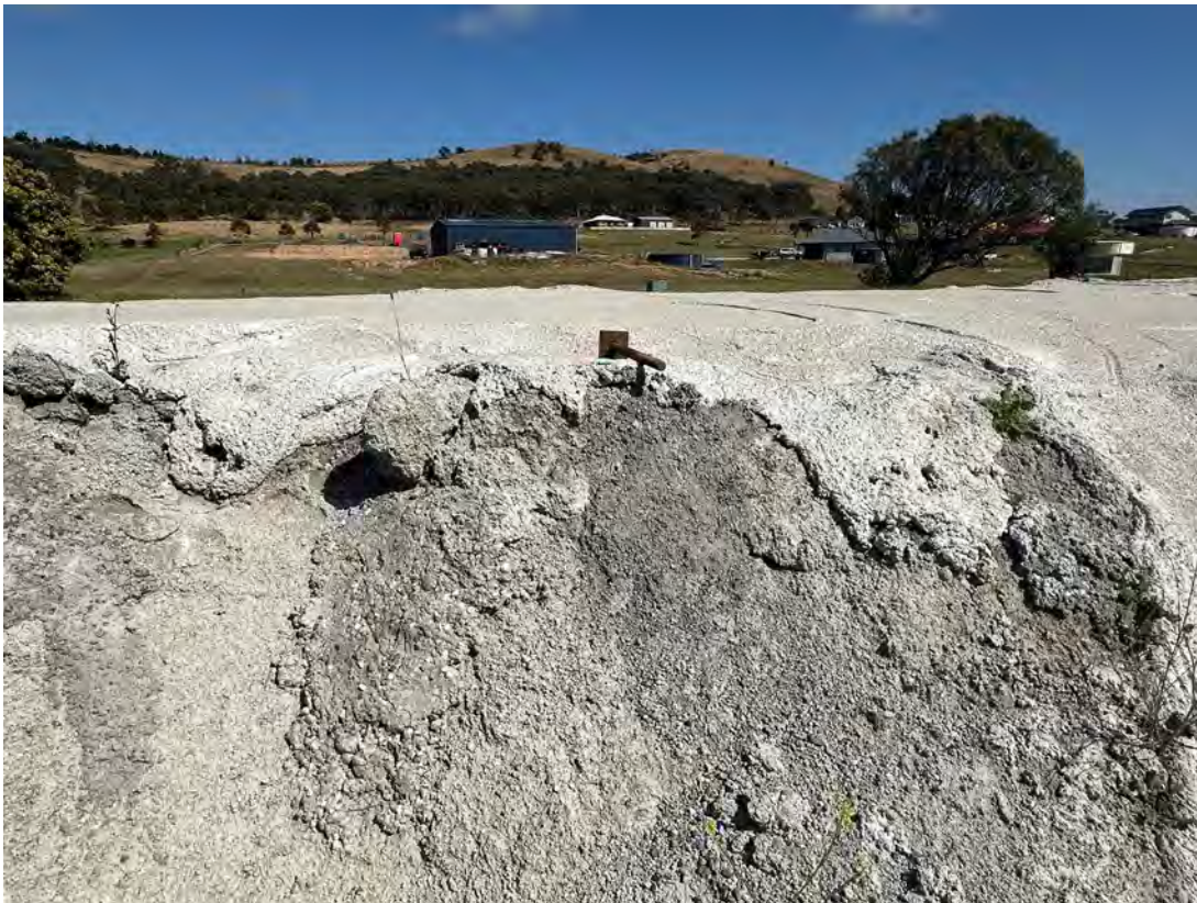
Photo 18: Exposed geofabric layer marker on stockpile identified in previous inspection has been filled with cement.
