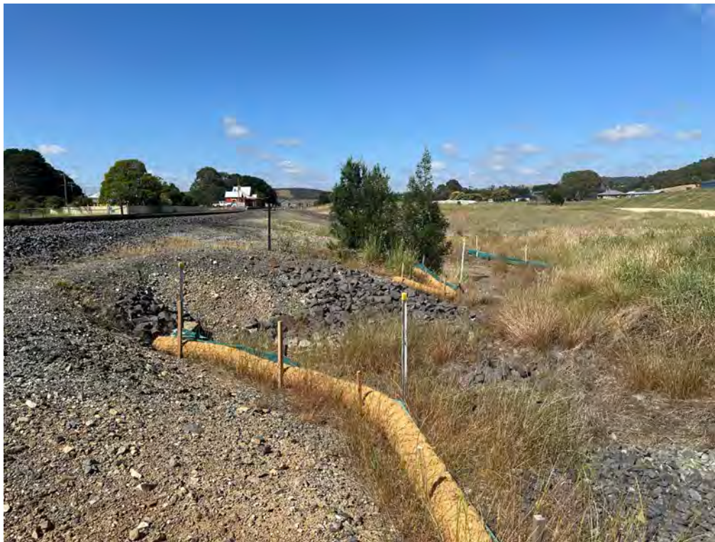
Photo 13: Upgradient of the railway line, north of the middle culvert, sediment coir logs in good condition. Minor inadequate ground cover observed during the previous inspections remained in a stable condition.
