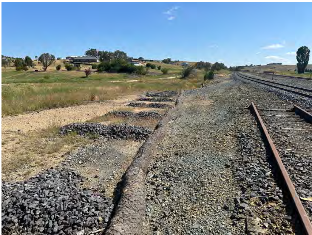
Photo 12: Rock armoury in drainage channel between southern and middle culverts appears to be in good condition.
