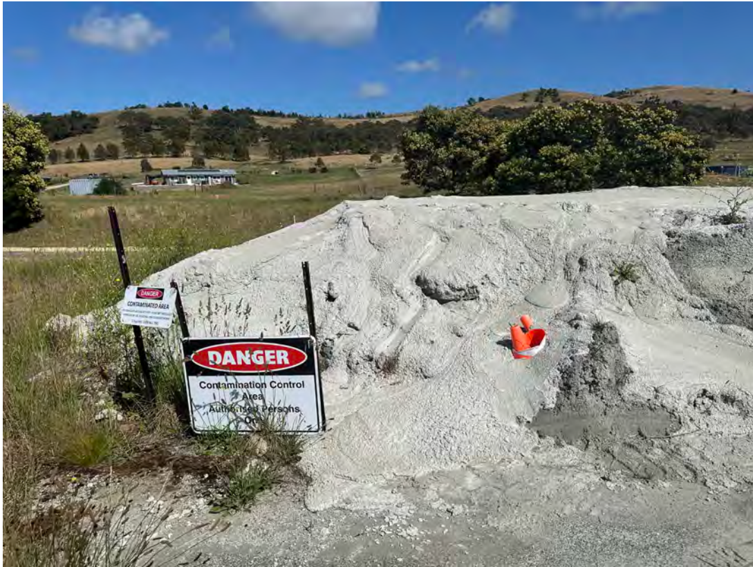
Photo 17: The concrete-capped stockpile is generally in good condition with no new erosion observed.
