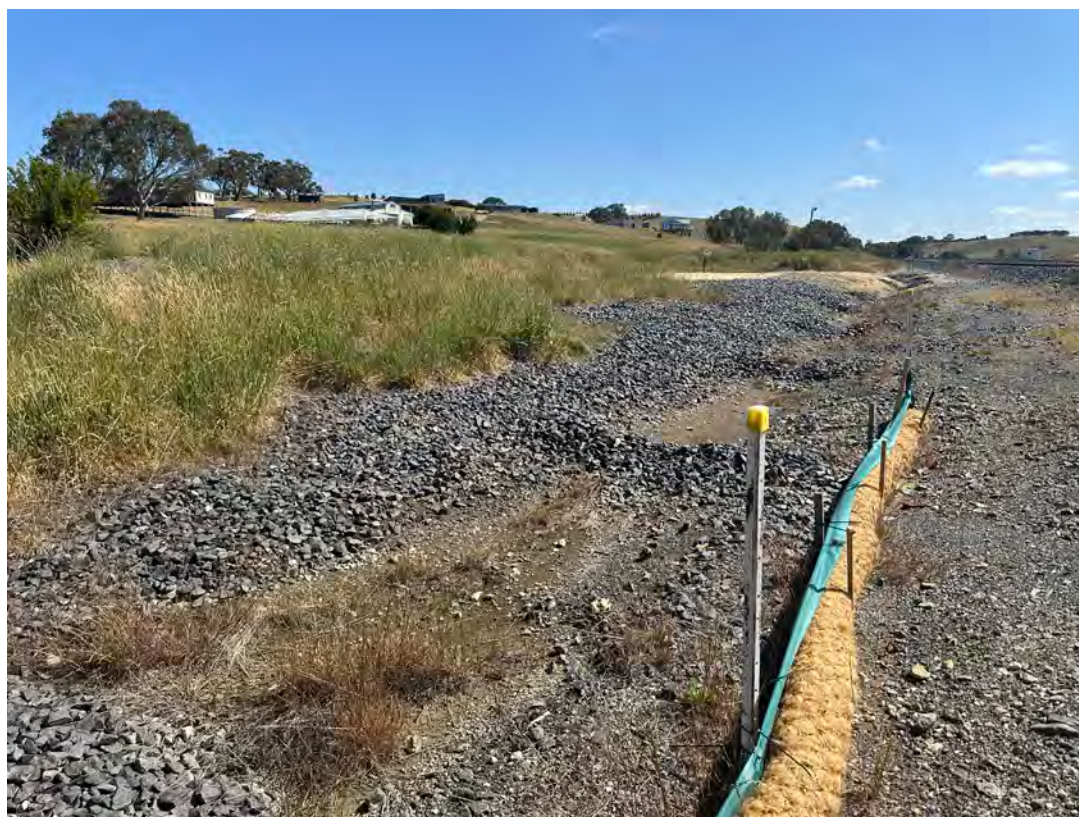
Photo 14: Rock armoury and sediment coir logs in drainage channel between middle and northern culverts appears to be in good condition.
