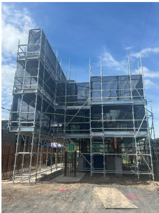
Scaffolding for Platform 2 lift construction.
