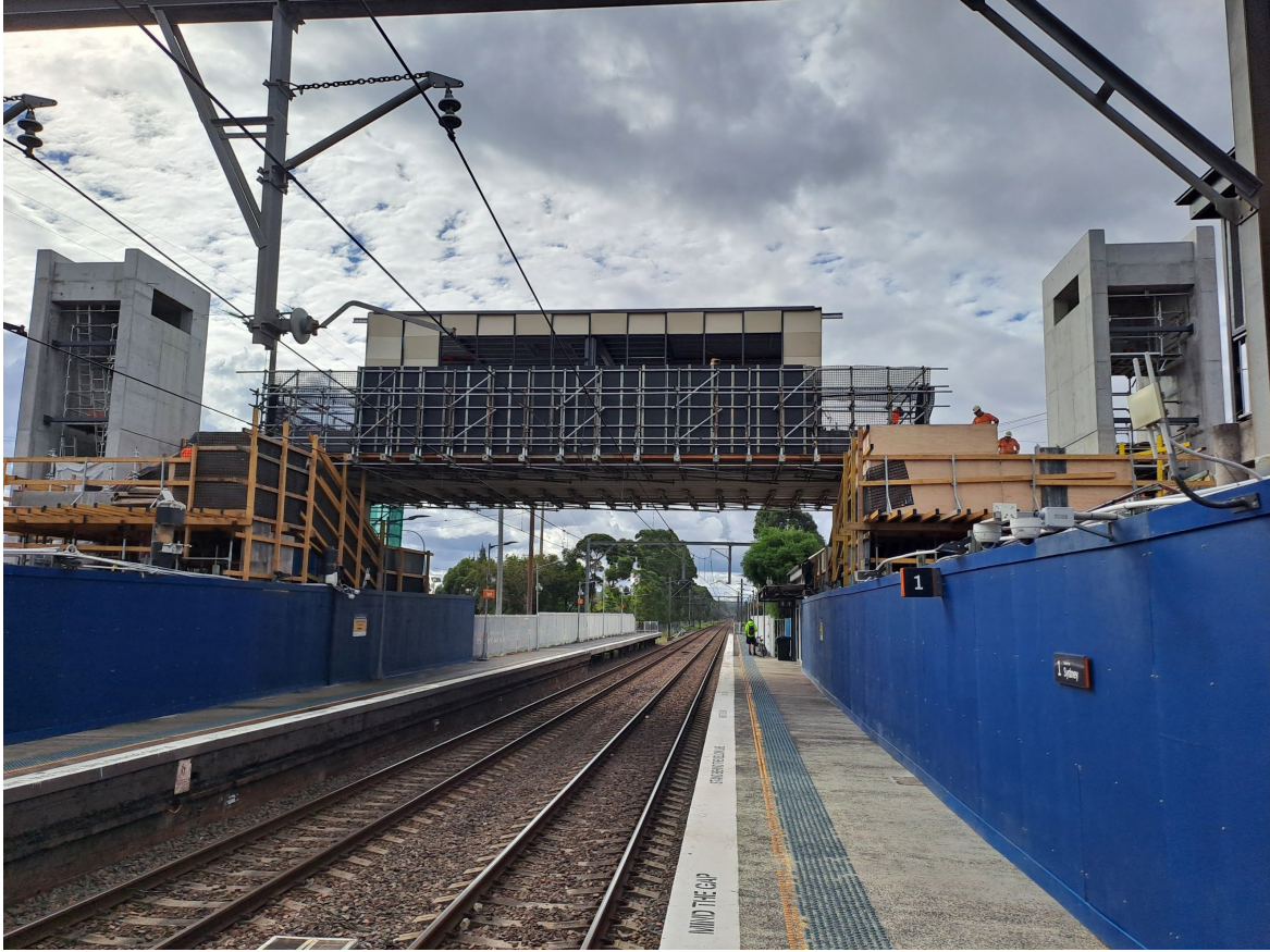
New pedestrian footbridge and lifts being constructed.
