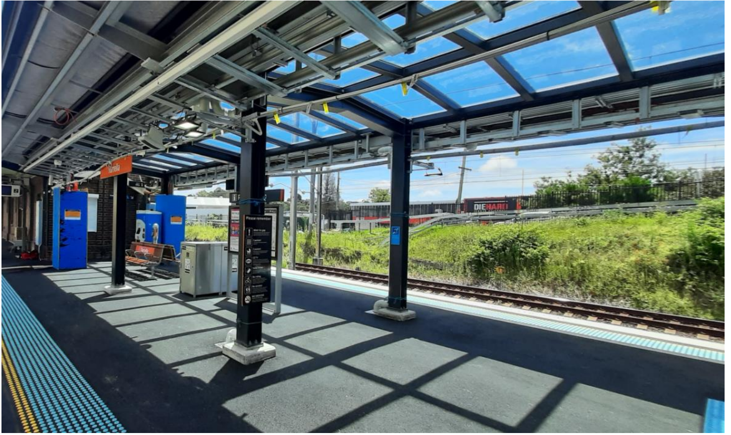
Image: Progress update of the platform canopy roof.
