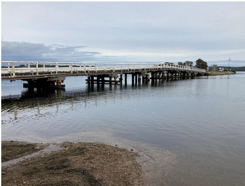
Wallaga Lake Bridge – View looking towards the Bermagui abutment
