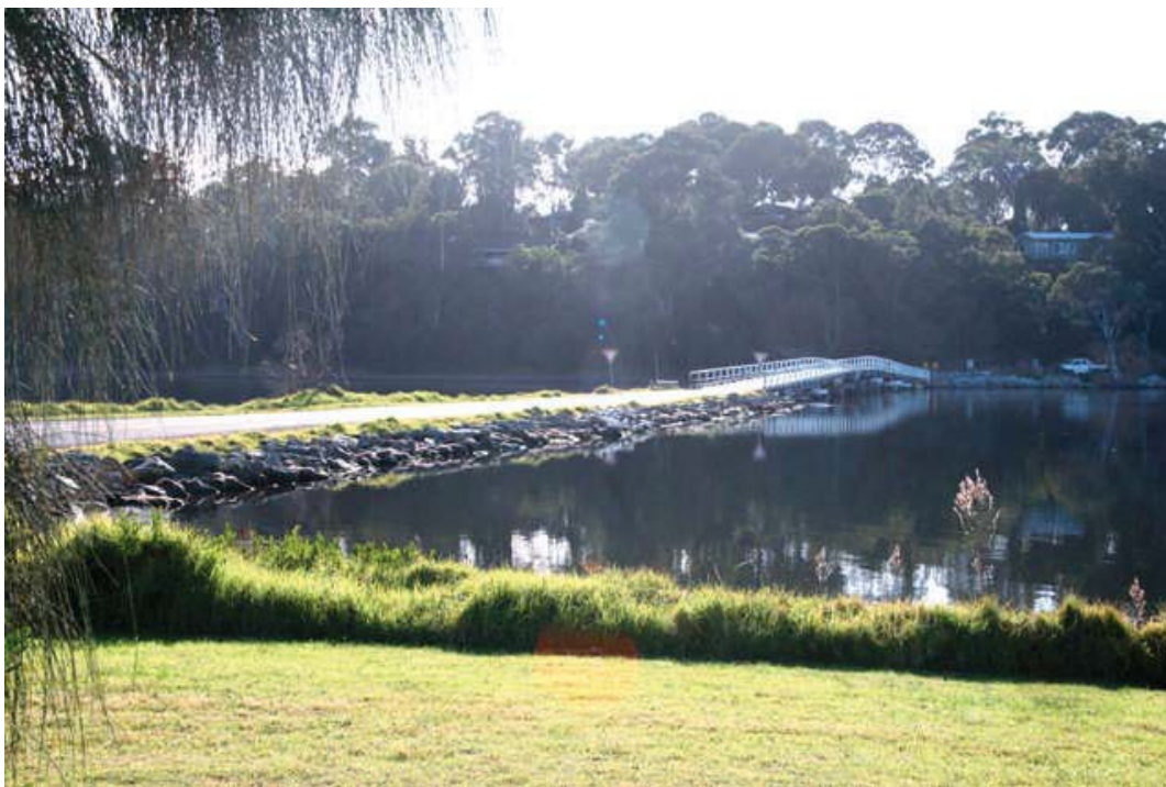
Figure 3: View looking north showing causeway and bridge.
