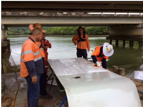
Figure 8a: Laminate being cut to size- note while white is shown, grey would be used at Wallaga Lakes Bridge. Figure 8b: Side and top views of works once completed.
