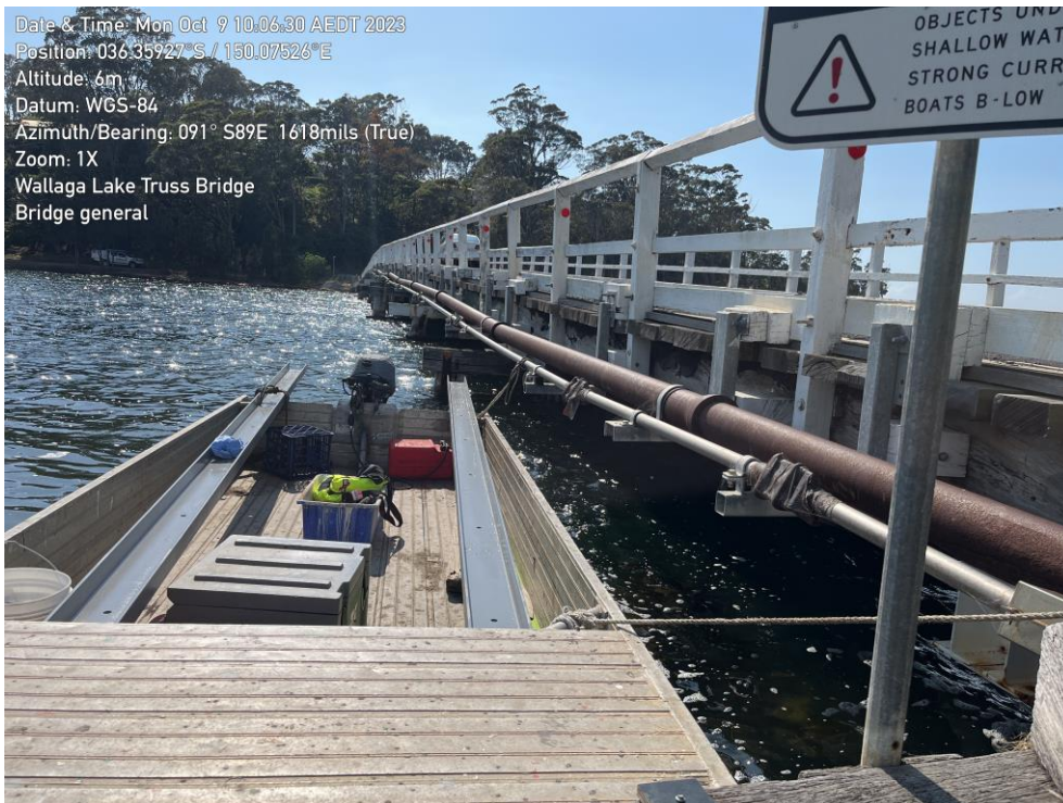
Figure 3-10: Bega Council sewer and drinking water lines
