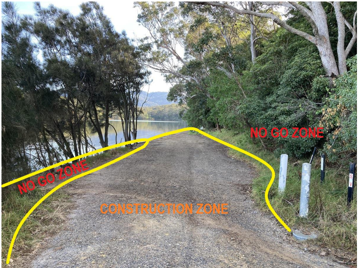
Figure 6-18: No-go areas on the left side of northern abutment
