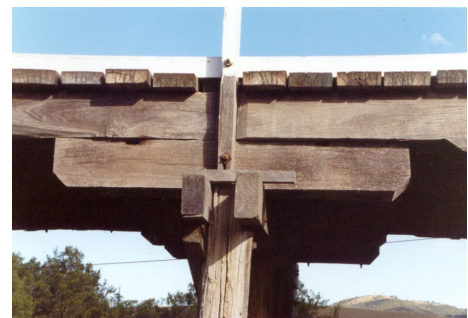
Figure 5a: Typical arrangement of a post-1894 timber beam design detailing the bridge components described in the text. Figure 5b: Allan's improved headstock design featuring two capwales.
