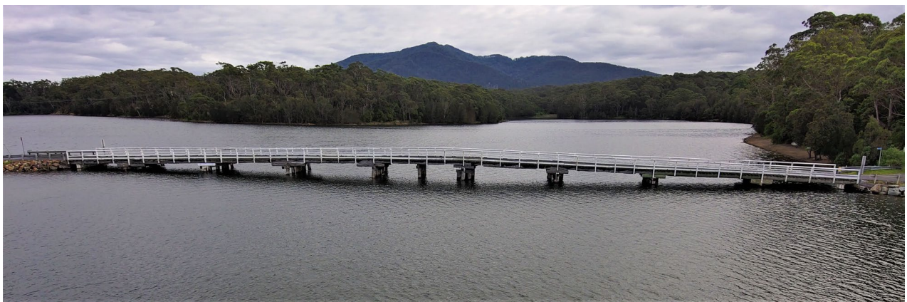
Figure 1: Profile view of bridge structure looking west in 2020.
