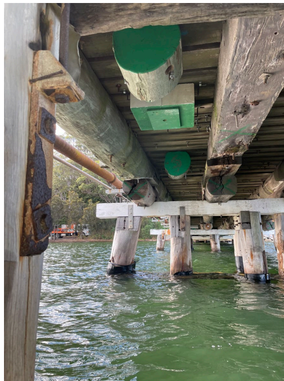
Figure 2-3: Example of Transport fabricated boxes – Timber and Hebel boxes.
