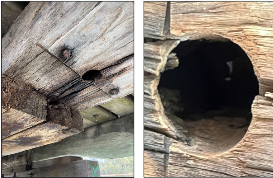
Figure 2-4: One of the exit locations within girder 19.
