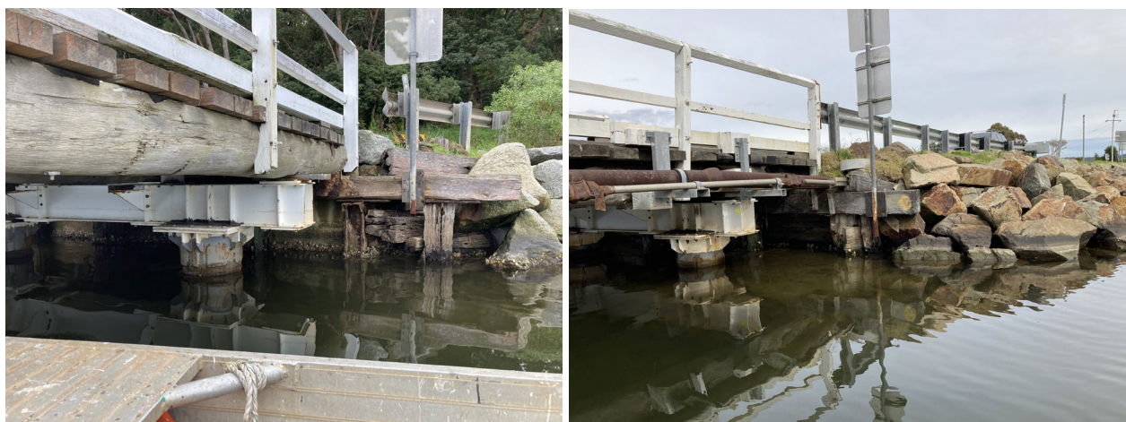
Figure 7a: Northern abutment face and eastern wingwall. Figure 7b: Southern abutment.
