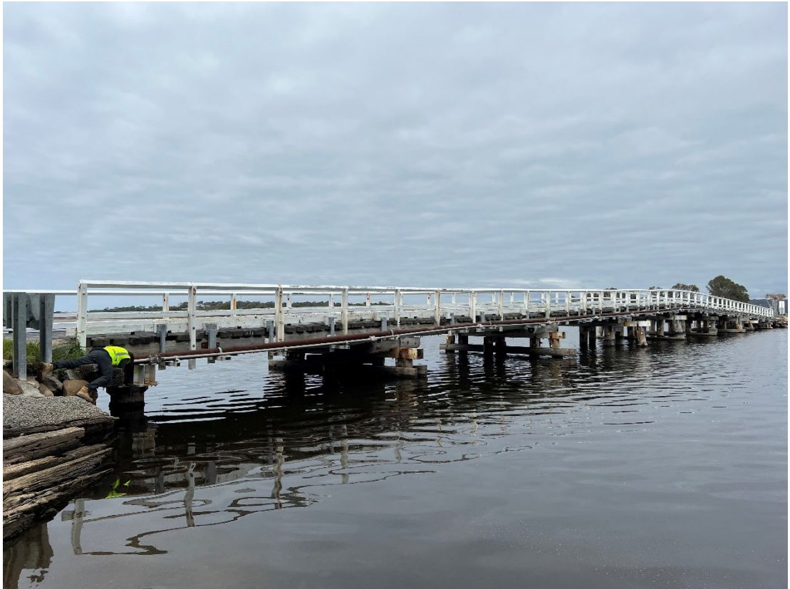
Figure 1-1: Wallaga Lake Bridge is a timber girder bridge.
