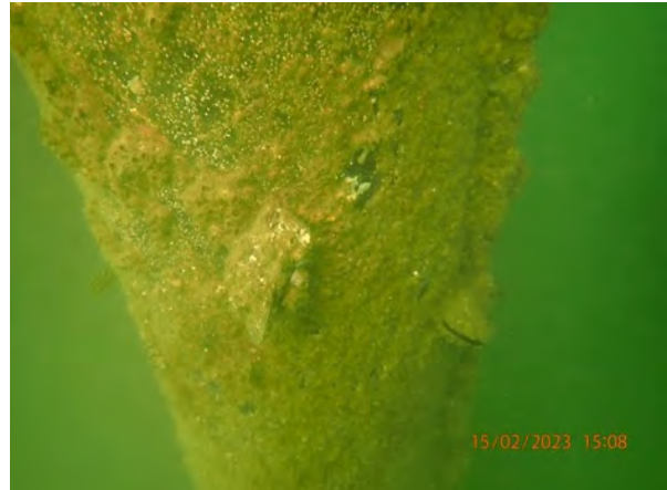
Photo 2. Typical pattern of marine growth on piles was limited to barnacles and mussels.
