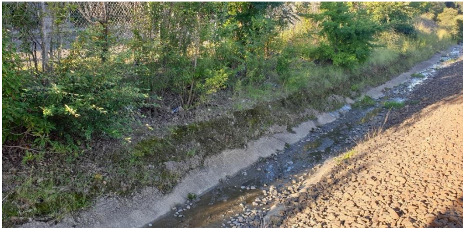
Photo 4: Small concrete drain on the up-side of the rail corridor
