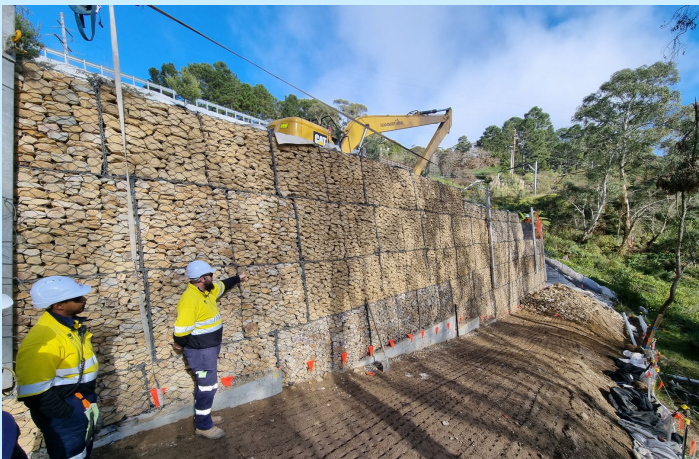
Constructing the gabion basket at Mount Victoria
