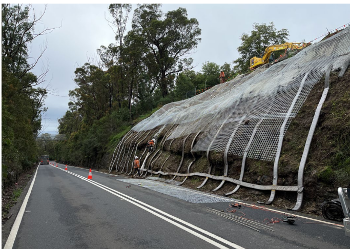
Wire mesh draping as part of emergency slope repair works on Bells Line of Road at Mount Tomah
