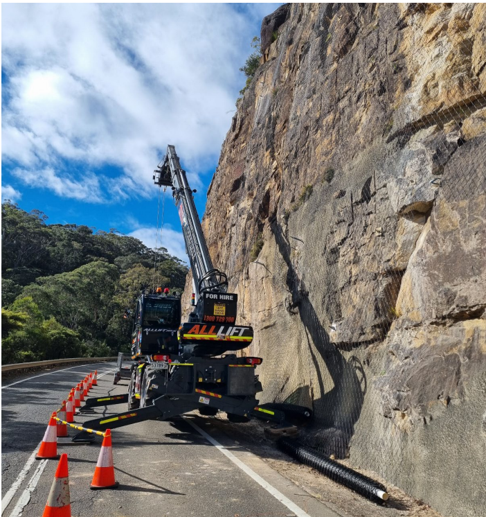
Installing wire mesh on Hawkesbury Road at Hawkesbury Heights
