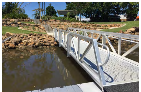
Figure 3 Pontoon and gangway installation with disability access ramp at Budd Park, Murwillumbah.
