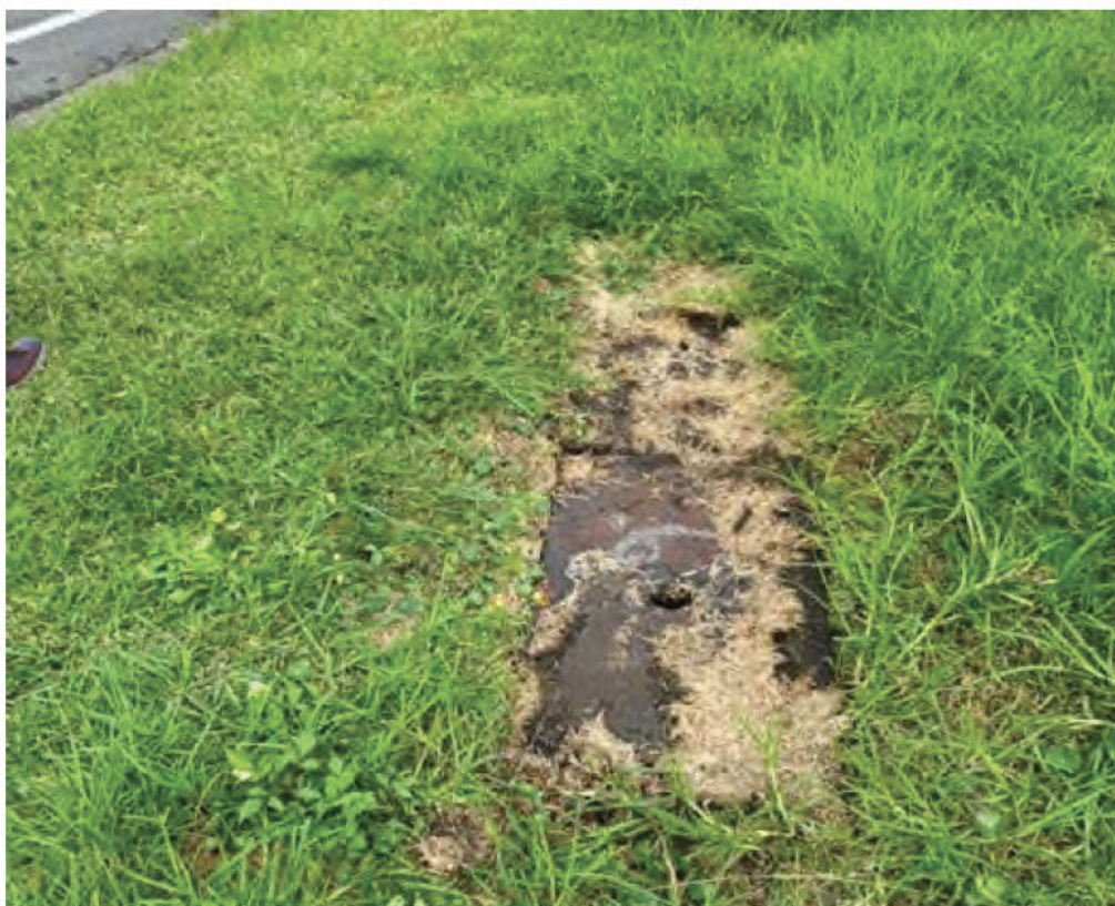
Figure 7: Existing asbestos pit to be removed (F)
