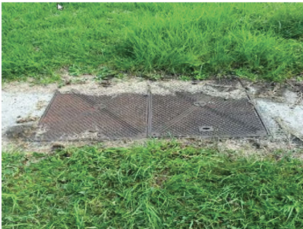
Figure 8: Existing manhole to be removed (E)
