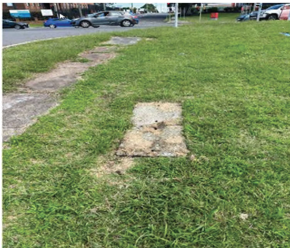
Figure 6: Existing pit (C) to be cut into
