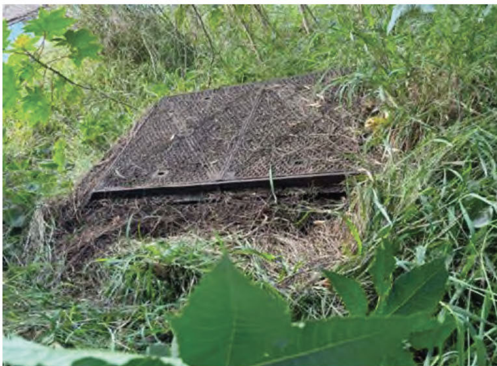
Figure 5: Existing manhole (A) to be accessed
