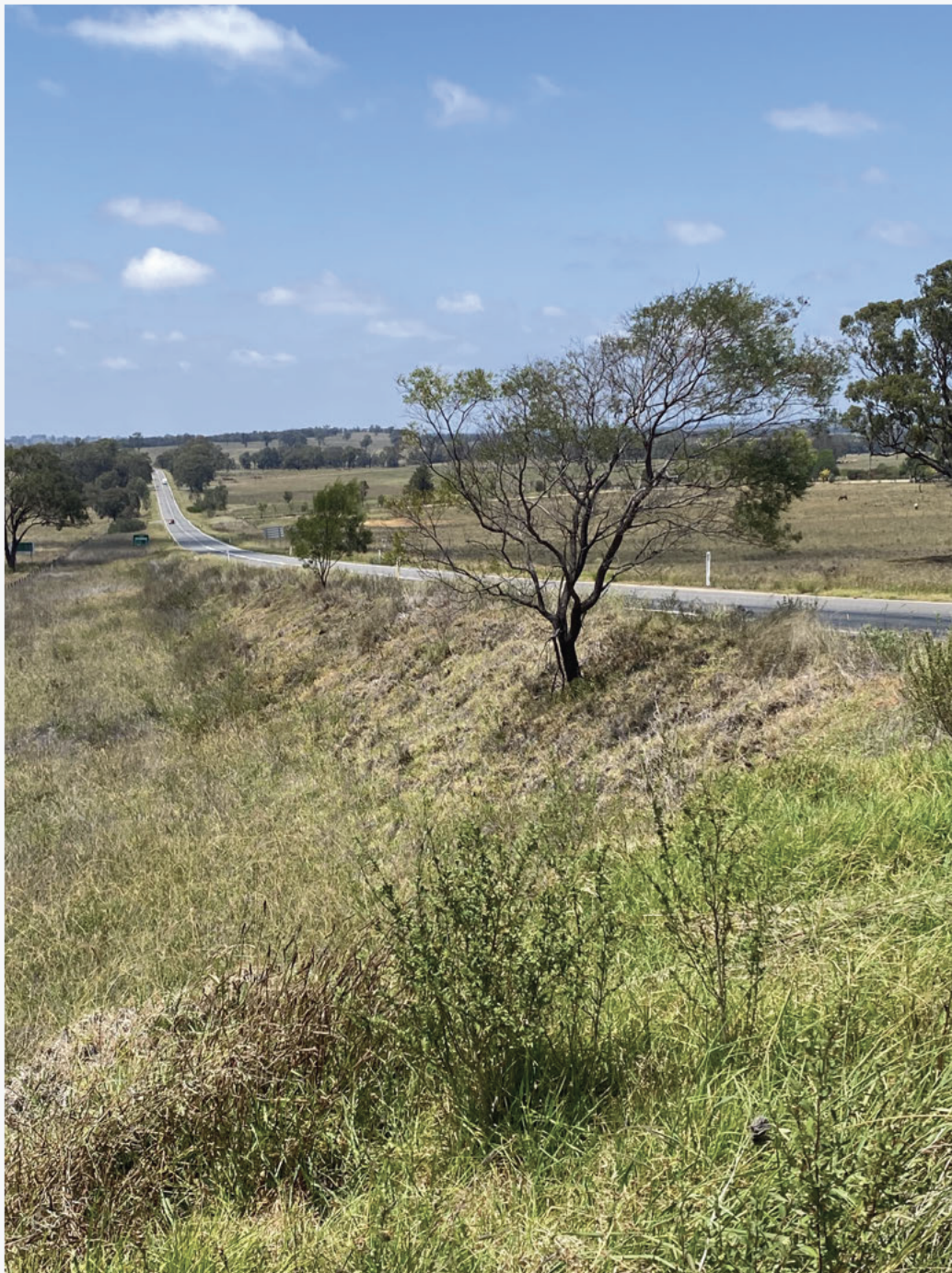
Figure 3-16: Site photograph of impacted tree – Golden Highway and Vinegaroy Road intersection (I-010)
