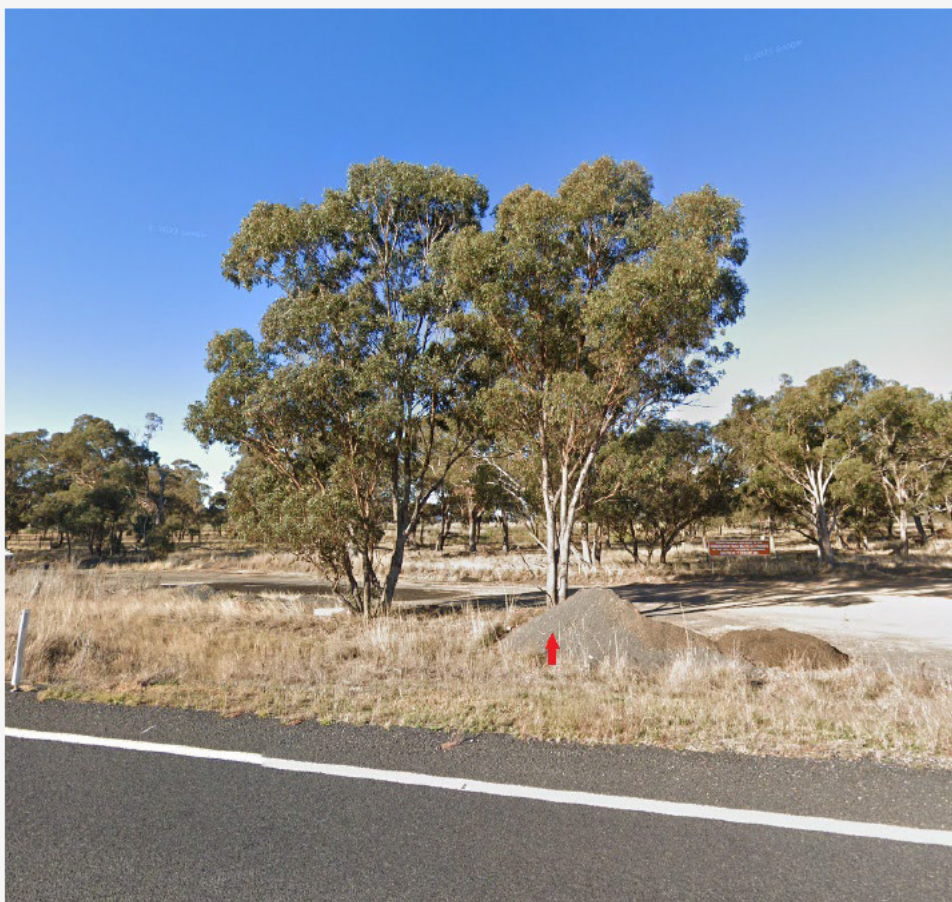
Figure 3-23: Tree removal potentially required on the eastern side of Castlereagh Highway, north of the Castlereagh Highway and Barneys Reef Road intersection for culvert replacement (Google Earth, 2023)
