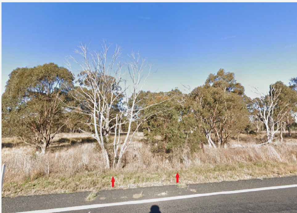
Figure 3-22: Tree removal required on the eastern side of Castlereagh Highway, south of the Castlereagh Highway and Barneys Reef Road intersection for culvert replacement (north of Figure 3-21) (Google Earth, 2023)
