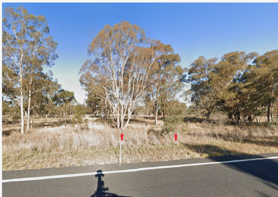
Figure 3-21: Tree removal required on the eastern side of Castlereagh Highway, south of the Castlereagh Highway and Barneys Reef Road intersection (southern end) for culvert replacement (Google Earth, 2023)
