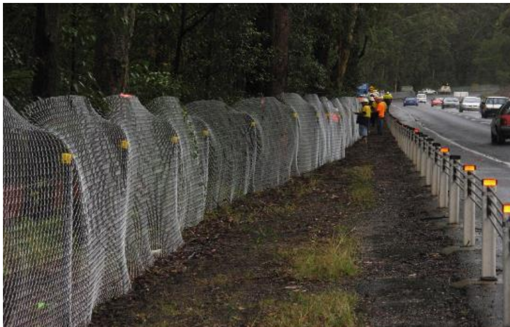
Figure 2.4: Example of temporary construction fauna exclusion fencing targeting koala on the Bonville Pacific Highway Upgrade Project (Photo: Scott Lawrence, TfNSW).
