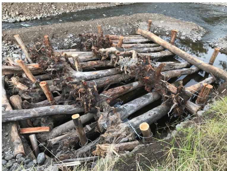
Figure 10.4: An Engineered Log Jam (ELJ) constructed using 'pin logs' and 'rootball logs' salvaged during clearing works creates aquatic habitat and protects from bank erosion achieving good river health outcomes (Photo: LLS).
