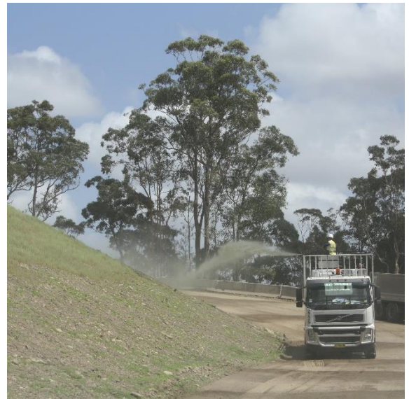
Figure 3.8: Hydromulch being sprayed on a batter on the Hunter Expressway (Photo: TfNSW).
