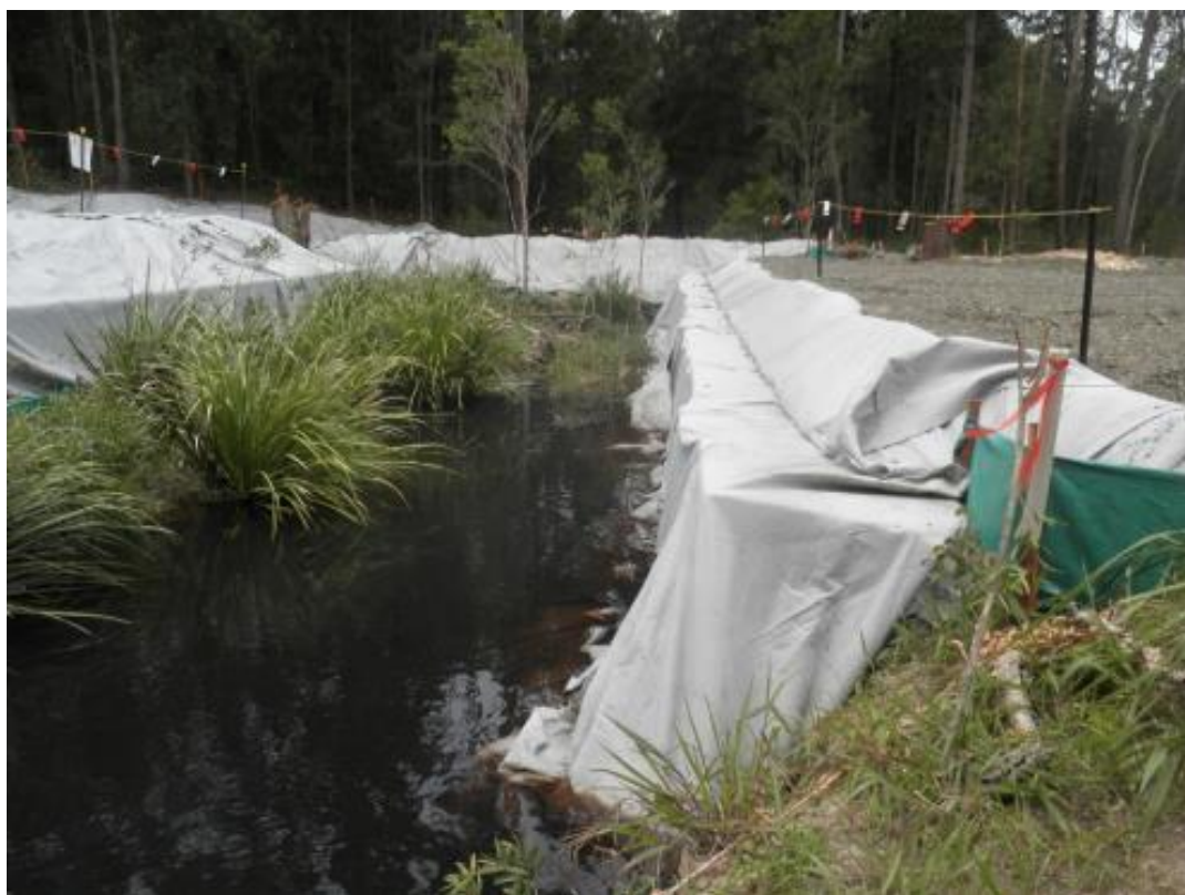
Figure 10.2: Working in riparian zones requires measures to protect the waterway, including geofabric to control erosion/sedimentation and exclusion fencing (Photo: TfNSW).
