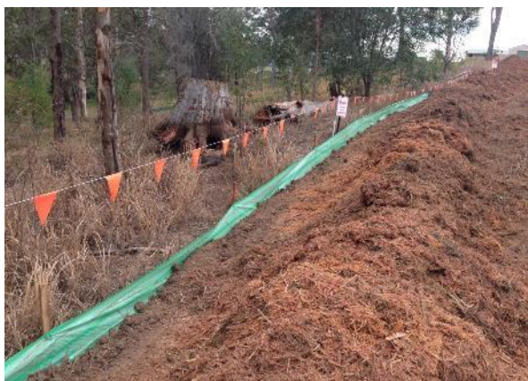
Figure 2.1: Example of mulch bund and construction flagging delineating the construction zone from the environmental protection area (Photo: Anthony Arena, TfNSW).
