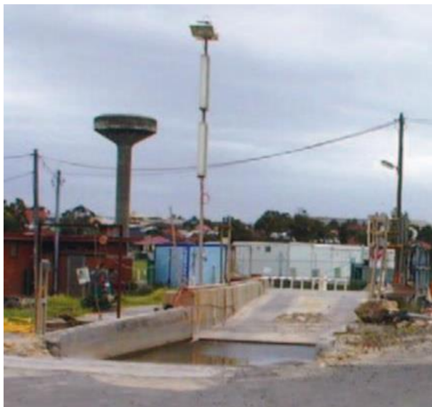
Figure 7.9: Wheel wash bay used at Tempe Reserve during construction of the Airport Link, Sydney Region. Most trucks drove through the wheel wash, but some vehicles needed to be scrubbed so that materials were not transported from site. The water depth was approximately 400mm, with a cattle grate underwater for solids to settle under (Photo: Leigh Trevitt, TfNSW).
