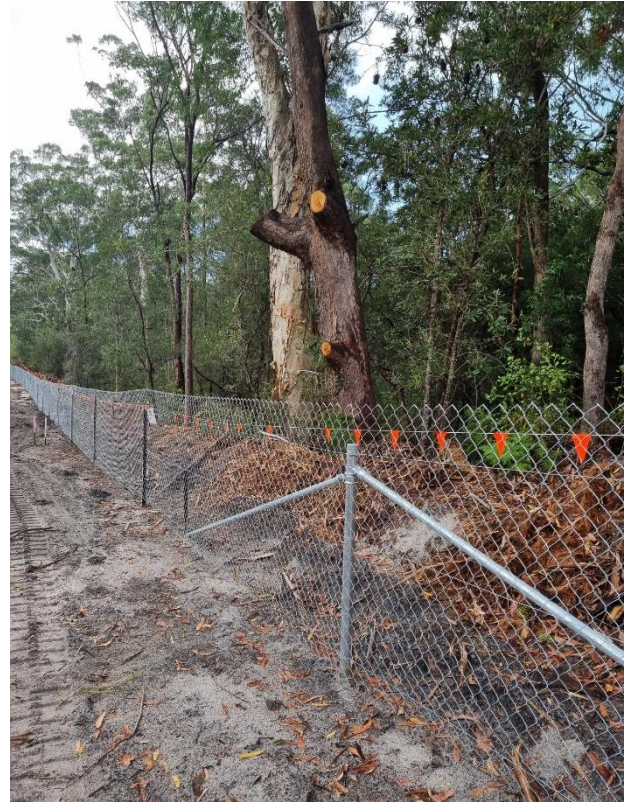
Figure 2.3: Example of temporary construction fauna exclusion fencing on the Nelson Bay Road Upgrade (Photo: Elle Hutchinson, TfNSW).
