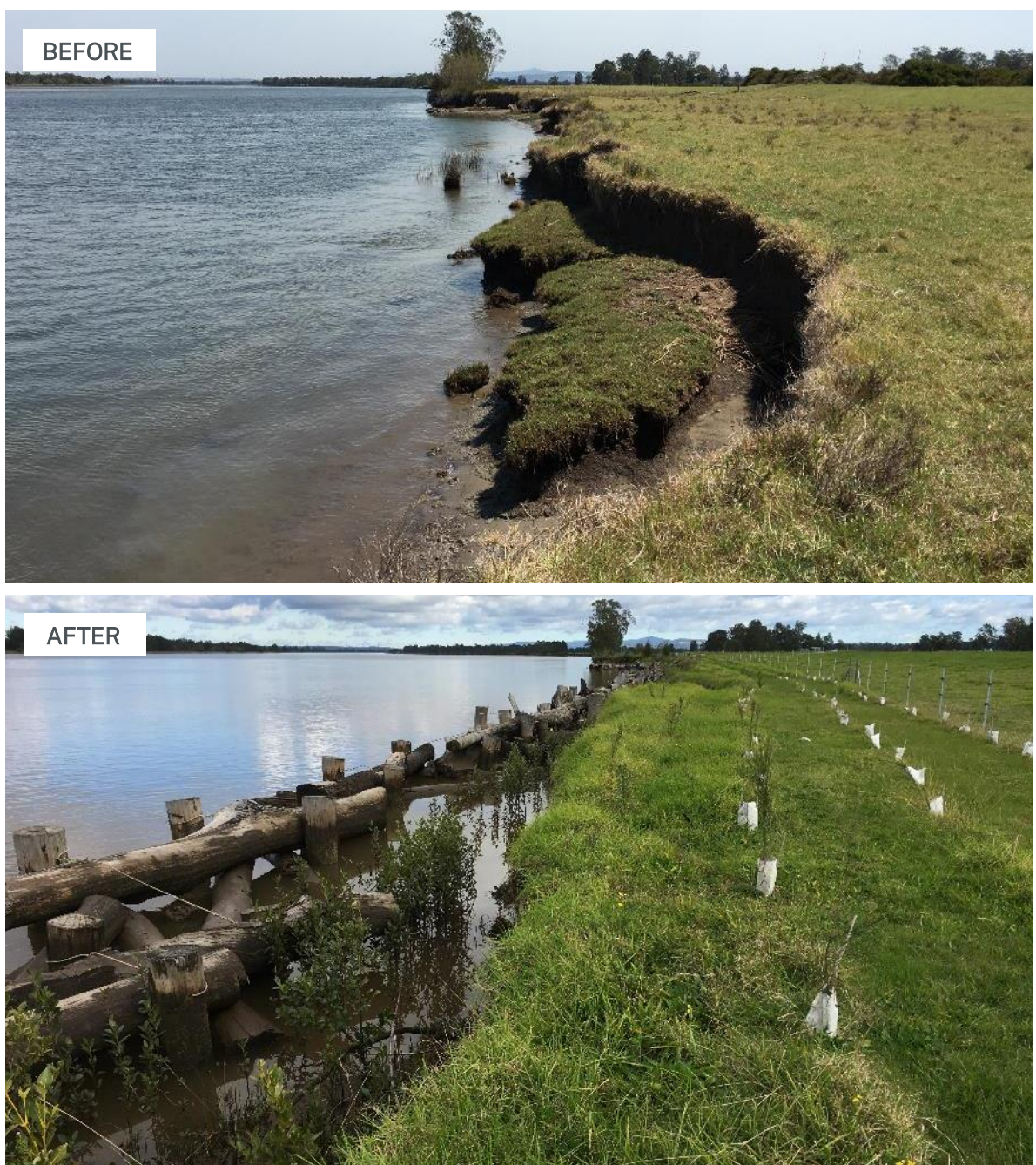
Figure 10.7: Before (above) and after (below) bank erosion management on the Hunter River at Millers Forest 2018-2020. Log walls were constructed from large woody debris salvaged during vegetation clearing (Photos: LLS).
