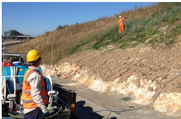
Figure 6.5: Herbicide application by foliar spraying on the Sapphire to Woolgoolga Pacific Highway Upgrade Project (Photo: Envite).
