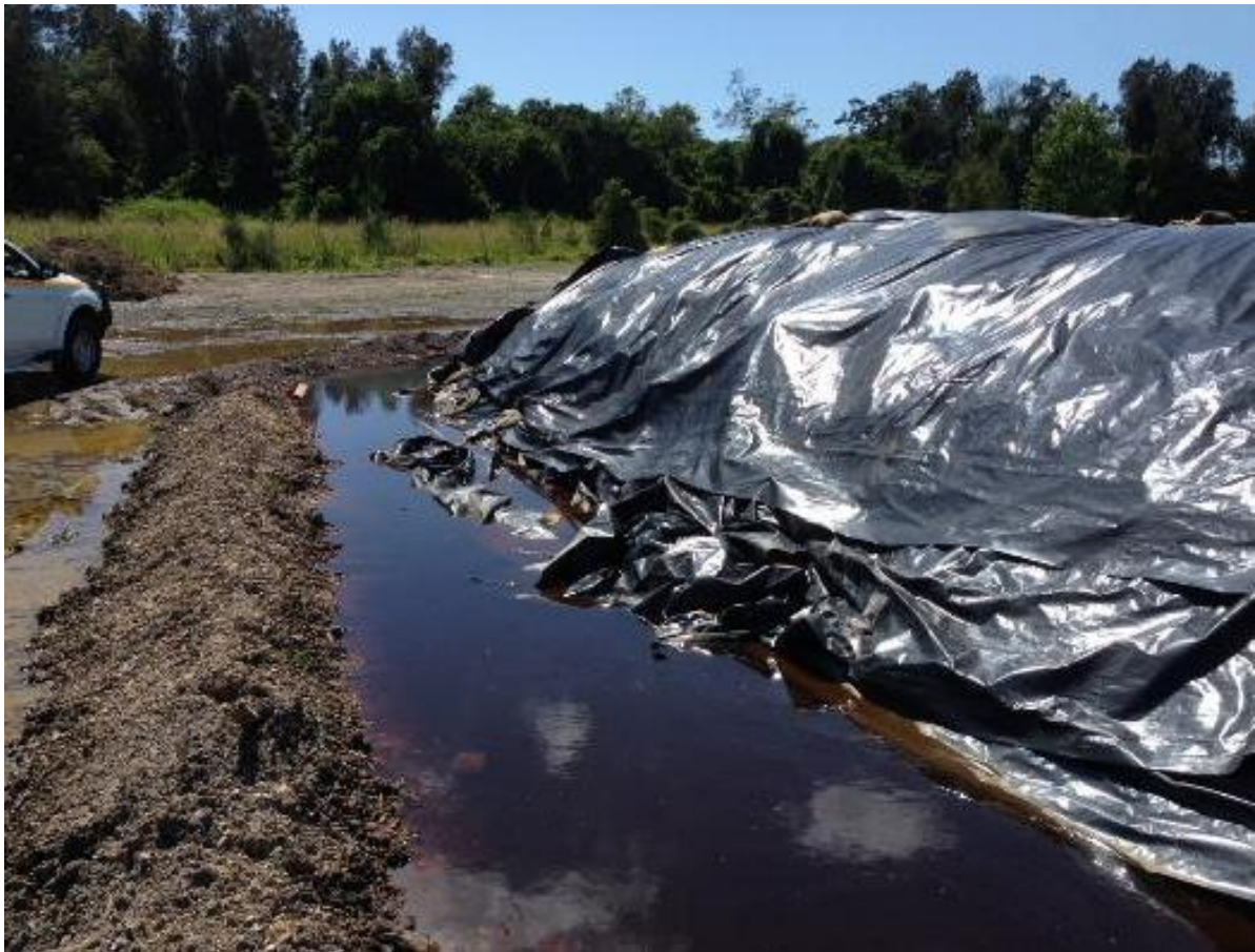
Figure 7.8: Soil solarisation to control soilborne pathogens using high temperatures on the Woolgoolga to Ballina Upgrade of the Pacific Highway) (Photo: Anthony Arena, TfNSW).
