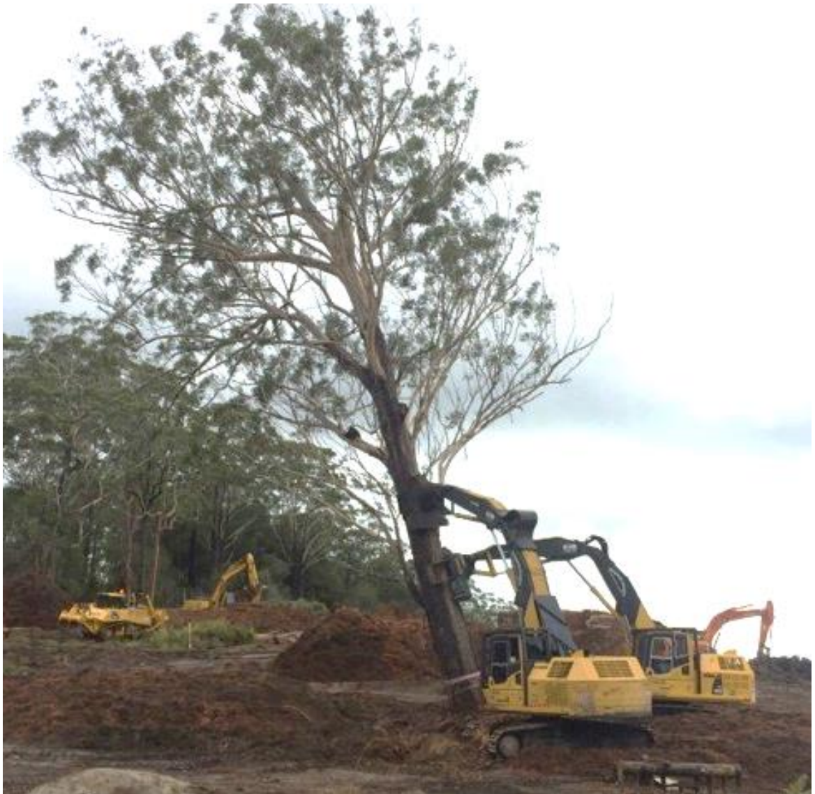
Figure 4.8: Habitat tree being carefully felled and lowered by excavators during the second stage of clearing for the Nambucca Heads to Urunga Pacific Highway Upgrade (Photo: Sandpiper Ecological Surveys).
