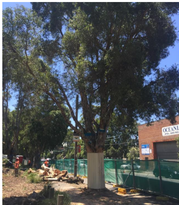
Figure 1.6: Tree-guards can be installed on trees during the pre-clearing process to prevent climbing animals being present during clearing (Photo: Brenton Hays, TfNSW)
