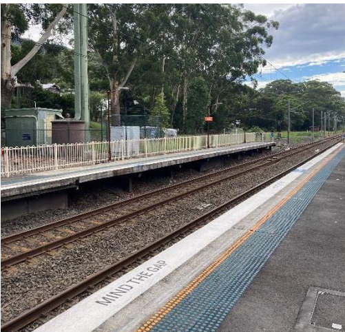
Figure 32: Photo of platform 1, showing the concrete supports of the platform, facing north
