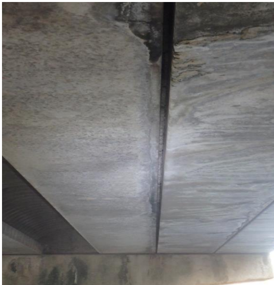
Expansion joint with staining from water leakage or microbat usage. Credit: Eco Logical
