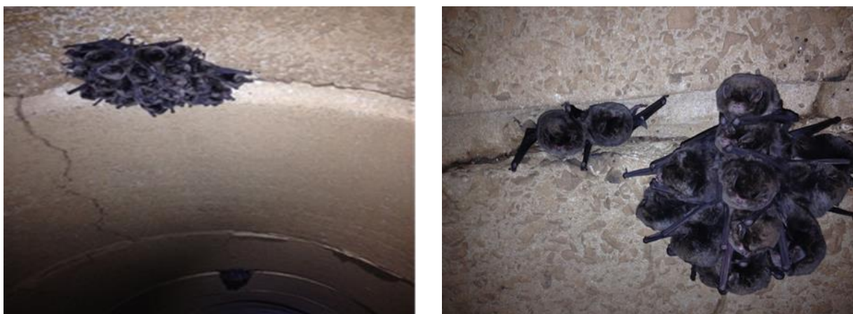
Known Southern Myotis breeding roost within unsealed joint gaps and voids within a 1200 mm 3-cell concrete pipe culvert. Credit: Veronica Silver, GeoLINK.
