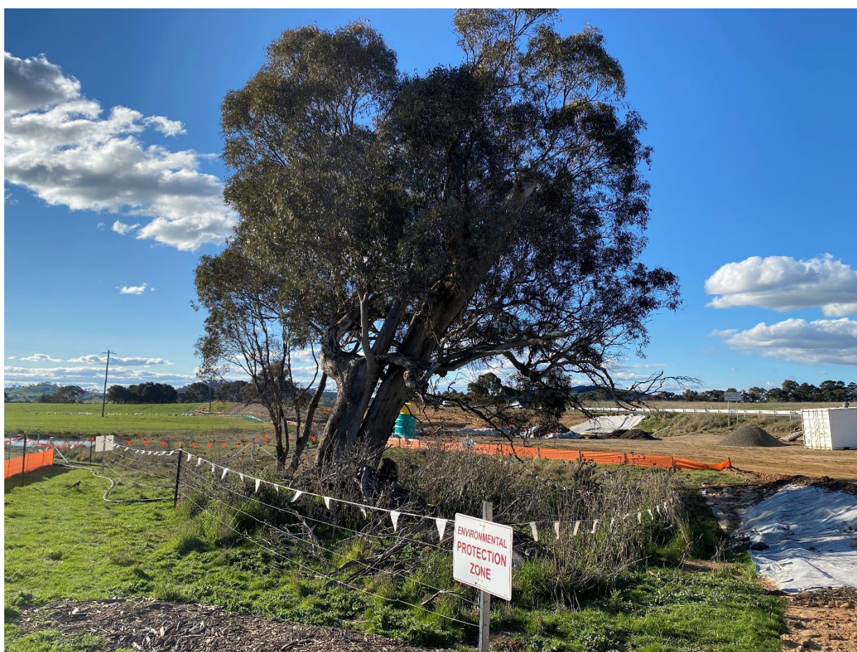
Figure 2.9: An example of tree protection using flagging on Barton Highway project (Photo: Amy Evans, TfNSW).
