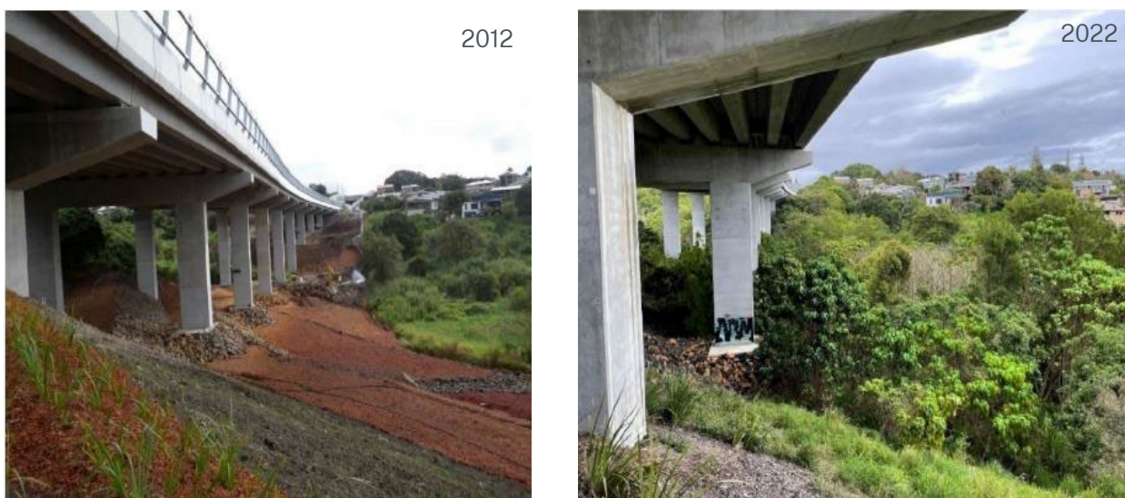
Figure 3.11: Ten years of rainforest revegetation, Banora Point Upgrade of the Pacific Highway. Photo on left taken post construction in 2012. Photo on right taken in 2022 showing progress over 10 year period (Photo: Alex Nicol, TfNSW).
