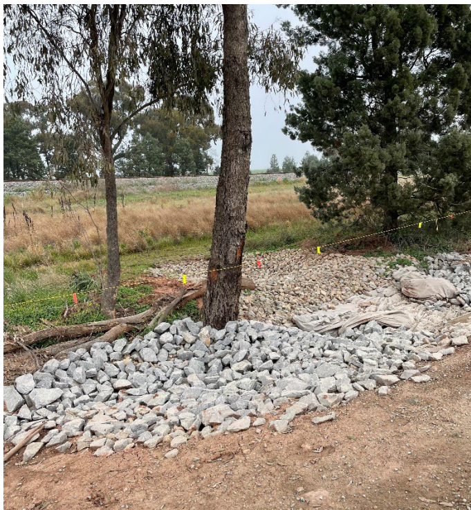
Figure 2.13: An example of poor practice. Construction materials should not be piled against trees and should be located outside the tree protection zone (Photo: Mel Cotterill, TfNSW).
