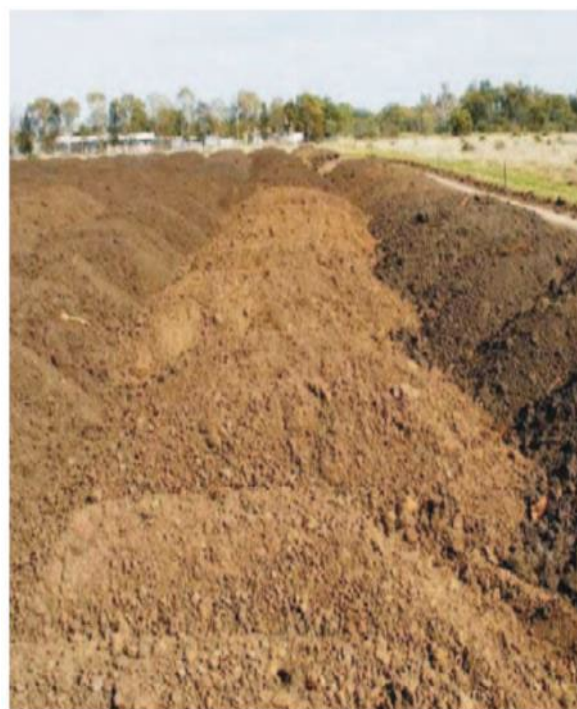
Figure 3.3: Topsoil being stockpiled at Moree for re-use later in revegetation and landscaping works (Photo: Lester Piggott, TfNSW).
