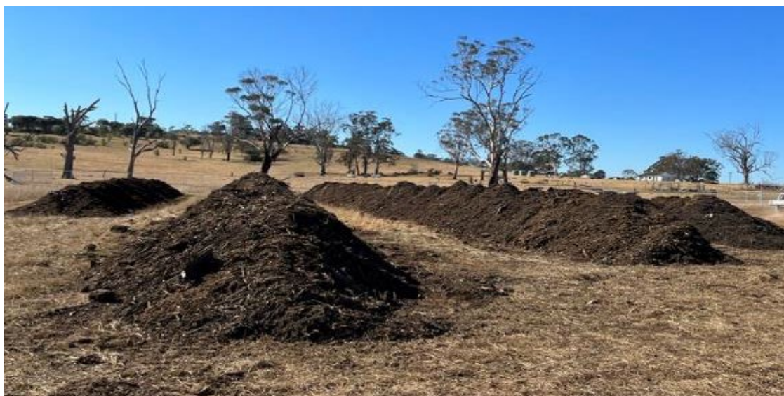
Figure 6.6: Windrows of weed-contaminated mulch are composted onsite for the Spring Farm Parkway Stage 1 Project. Composting creates high temperatures that can destroy organic toxins, weeds seeds and plant propagules and disease organisms (Photo: Amanda Berger, TfNSW).
