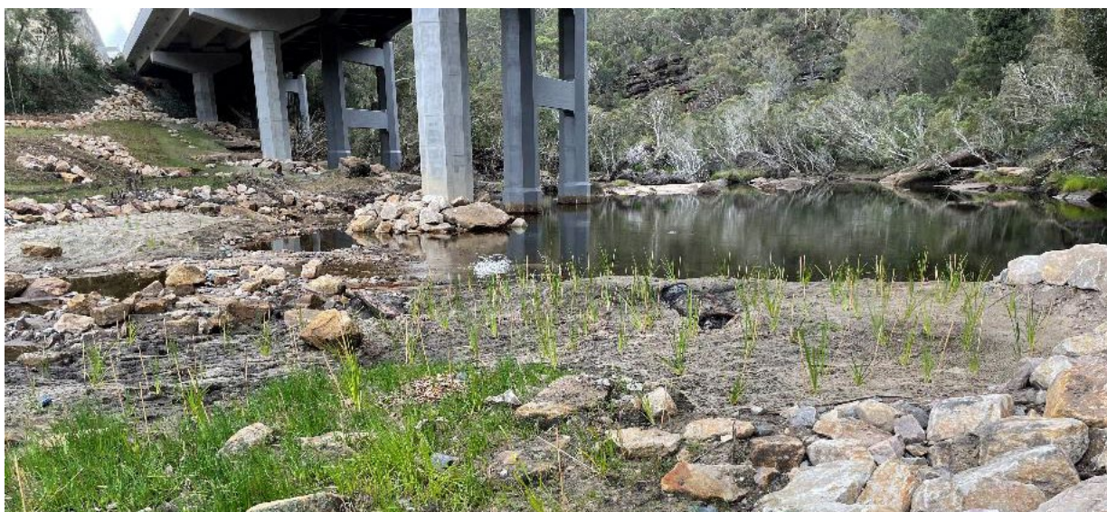
Figure 10.6: Planting wetland species and placement of rock within the Woronora River to reestablish aquatic habitats following completion of the Heathcote Road Bridge upgrade (Photo: Julie Ravallion, TfNSW).
