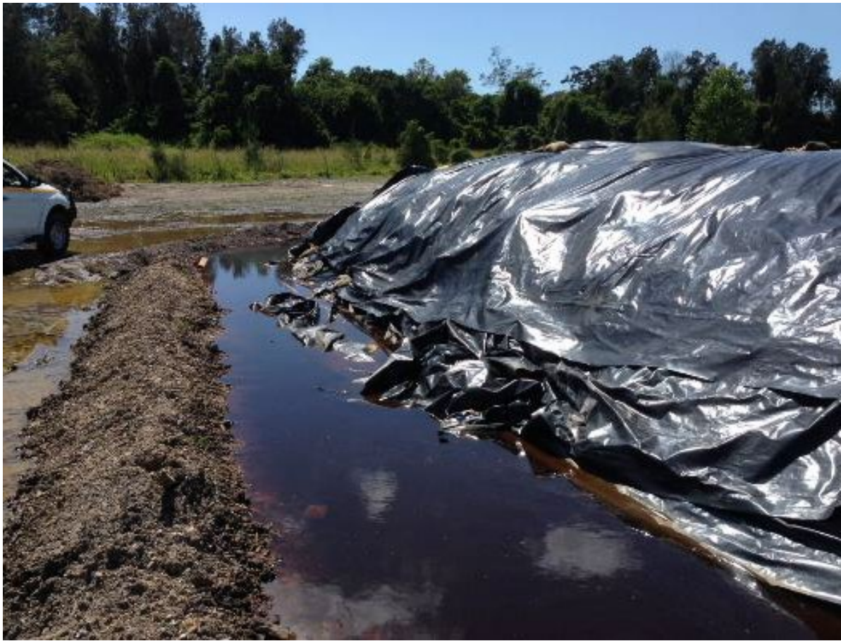
Figure 7.8: Soil solarisation to control soilborne pathogens using high temperatures on the Woolgoolga to Ballina Upgrade of the Pacific Highway) (Photo: Anthony Arena, TfNSW).
