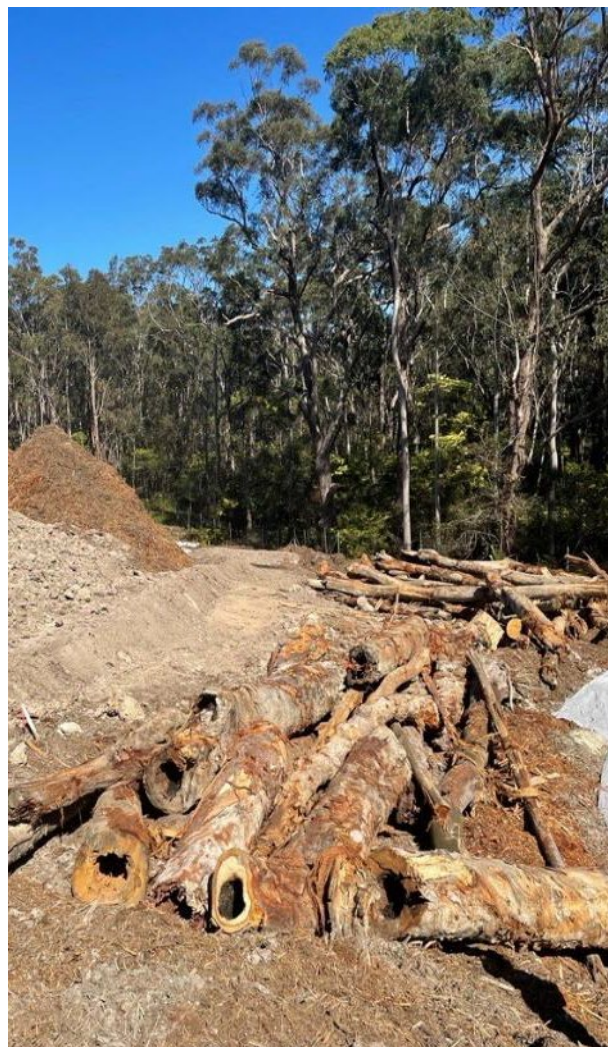
Figure 5.3: Hollow logs retained during clearing and stockpiled for relocation as fauna habitat on the Rankin Park to Jesmond Inner-city Bypass Project (Photo: Rebecca Vaughan, TfNSW).
