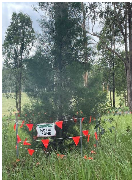
Figure 2.2: Exclusion fencing around a retained threatened Bailey's Cypress Pines ( Callitris baileyi ) on the Bruxner Highway (Photo: Ben Christiansen, TfNSW).
