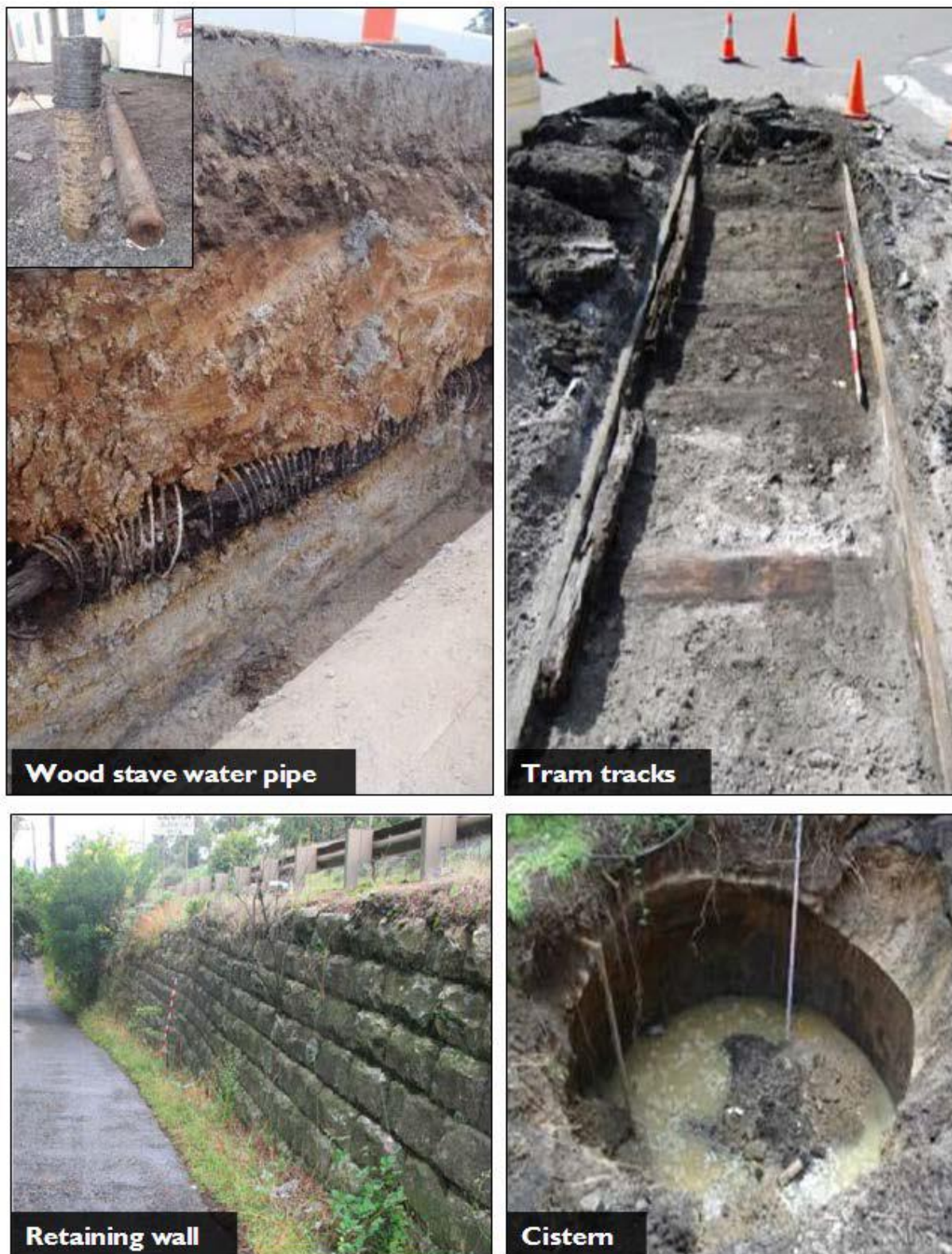
Figures: Top left hand picture continuing clockwise: woodstave water pipe with tar and wire sealing (Horsley drive); tram tracks (Sydney); brick lined cistern (Clyde); retaining wall (Great Western Highway, Leura).
