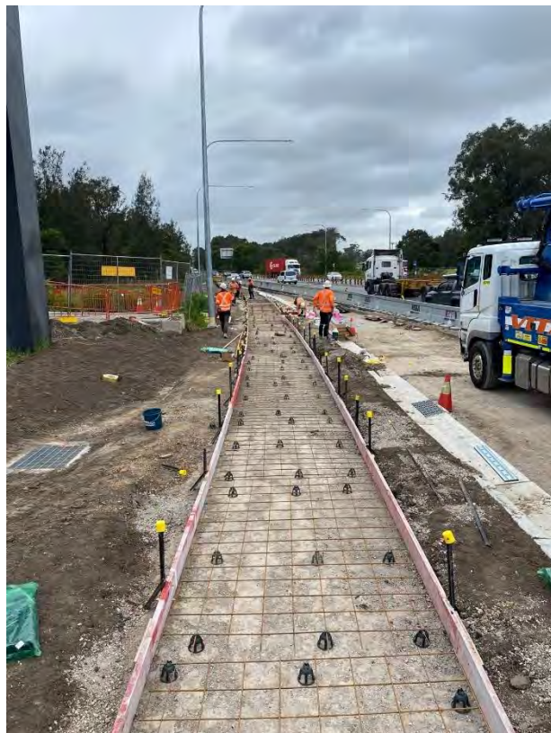
Pavement works along the slip lane from Henry Lawson Drive to Milperra Road.
