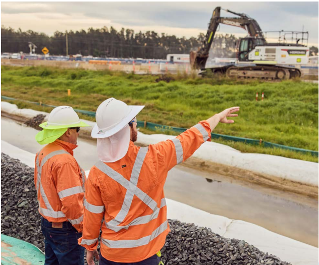
Field workers performing inspections of sediment control measures installed to protect waterways during construction of M1 Raymond Terrace extension
