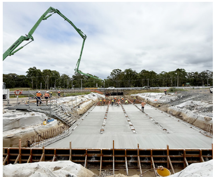
The largest concrete pour of the project at the upgraded culvert near Willowgreen Road.
