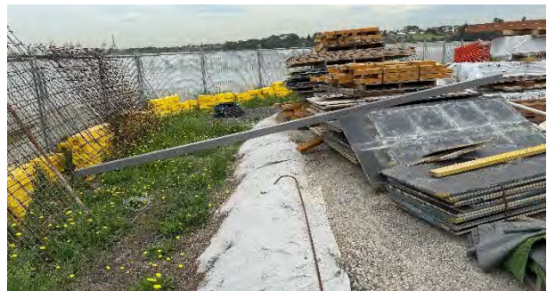
Photo LP3a and 3b: La Perouse site compound – Entire site compound lined with geofabric and road base to prevent disturbance of AHIMS Site# 45-6-0650 (Site 3 - La Perouse).
