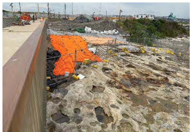
Photo LP7: Rock ballast removed to expose rock platform.
