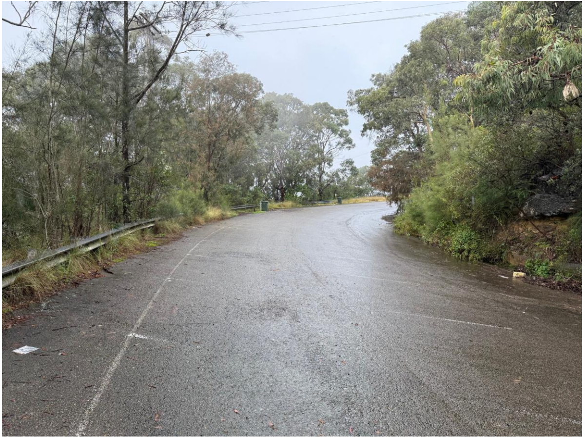
Figure 2-7: Image of site compound No.2
