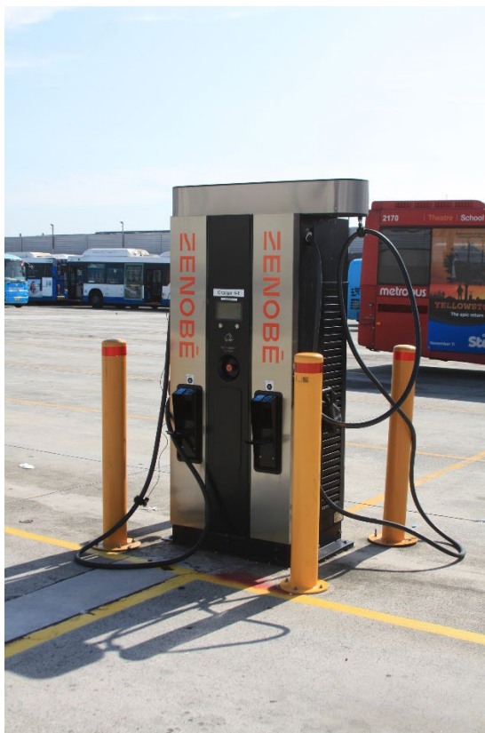
Existing charging plinths in the bus depot yard and surrounding deflection barriers (DC)
