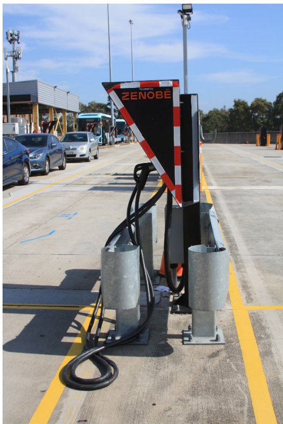
Existing charging plinths in the bus depot yard and surrounding three beam deflection barriers (AC)
