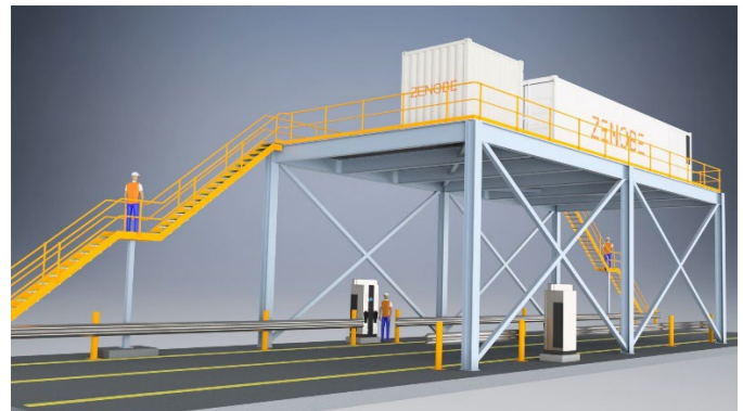
Figure 8 Additional visualisation of proposed raised cable containment culvert and shipping containers above it from ground level.
