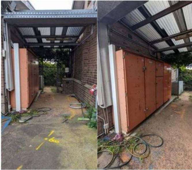
Figure 18 switch board attached to former SRA office and amenities building, facing west, note the existing connections into the building at the top and into the connections at the side. Connections also extend under the switchboard.
