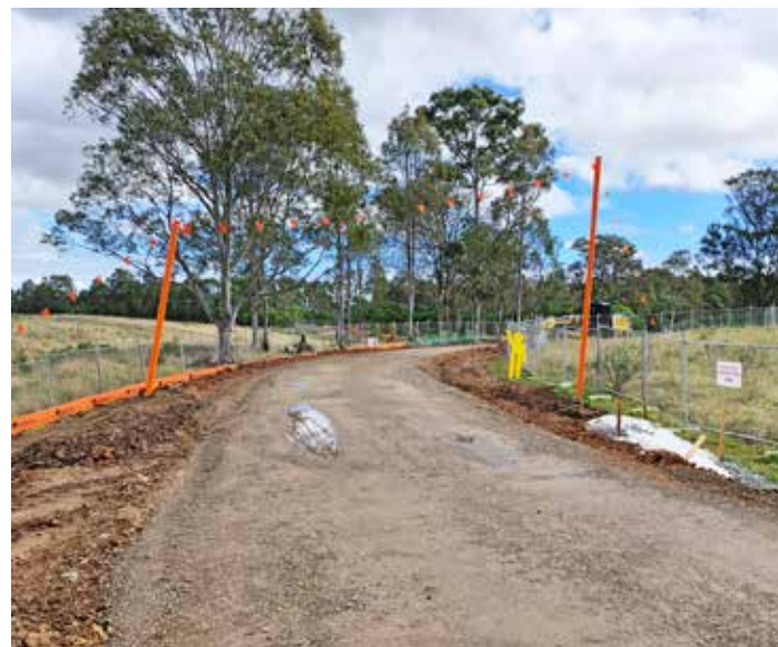
Building the new M7 to M12 shared path connection
