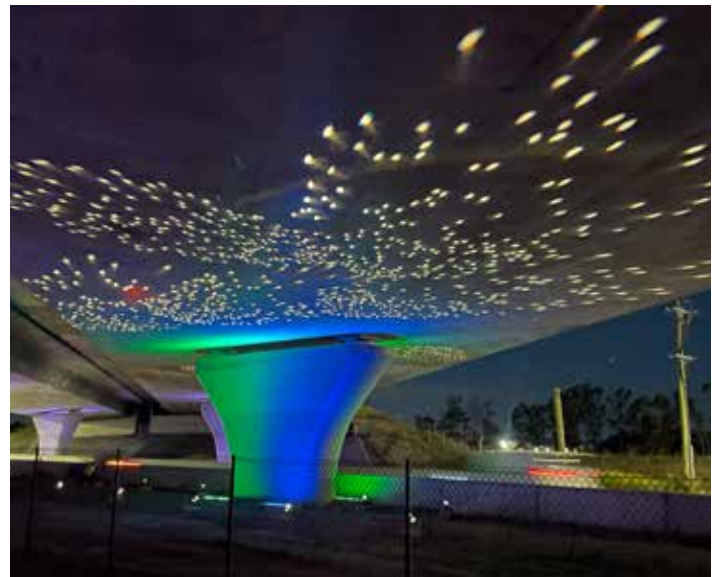
Let there be light: testing the new feature lights under the M12 Motorway bridge over Elizabeth Drive near Mamre Road
