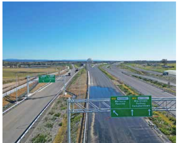
New road signs installed on Warami Drive, looking north
