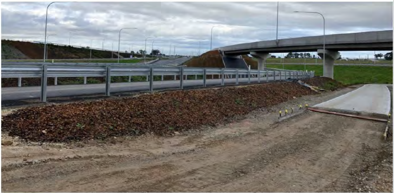
Earthen bund installed with active vehicle movements in this area whilst the Emu in the Sky continues to be constructed
