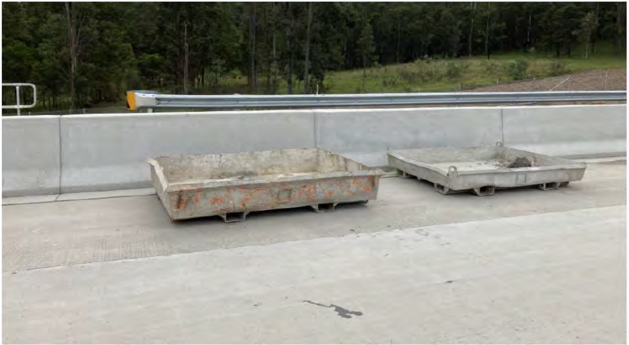
Concrete trays available for batter chute concrete pours
