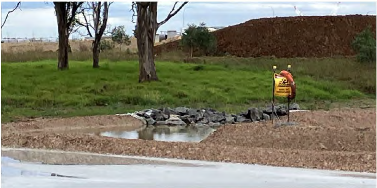
Overflow sump for slurry management with safety equipment available.
