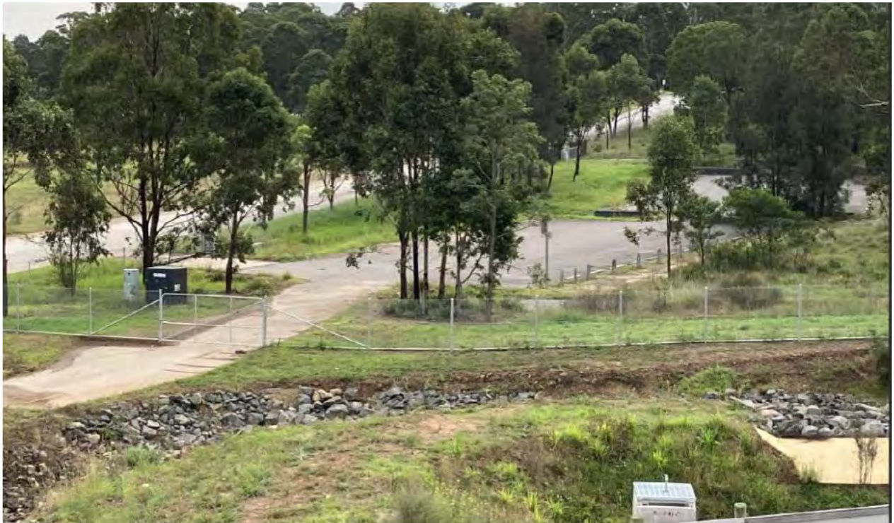
Former Range Road Ancillary Facility with rock lined swale installed.
