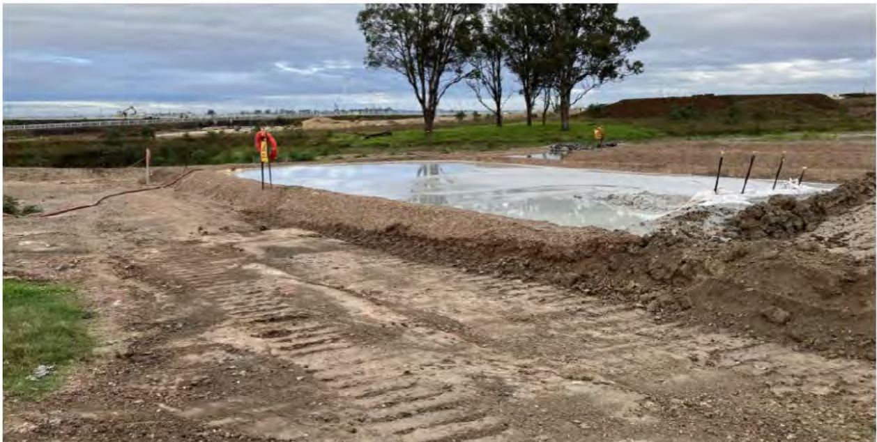
Basin for treatment of grinding and grooving slurry
