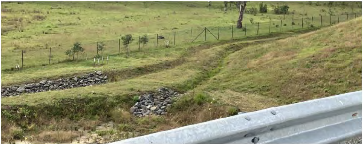
Grass lined swales with rock placement
