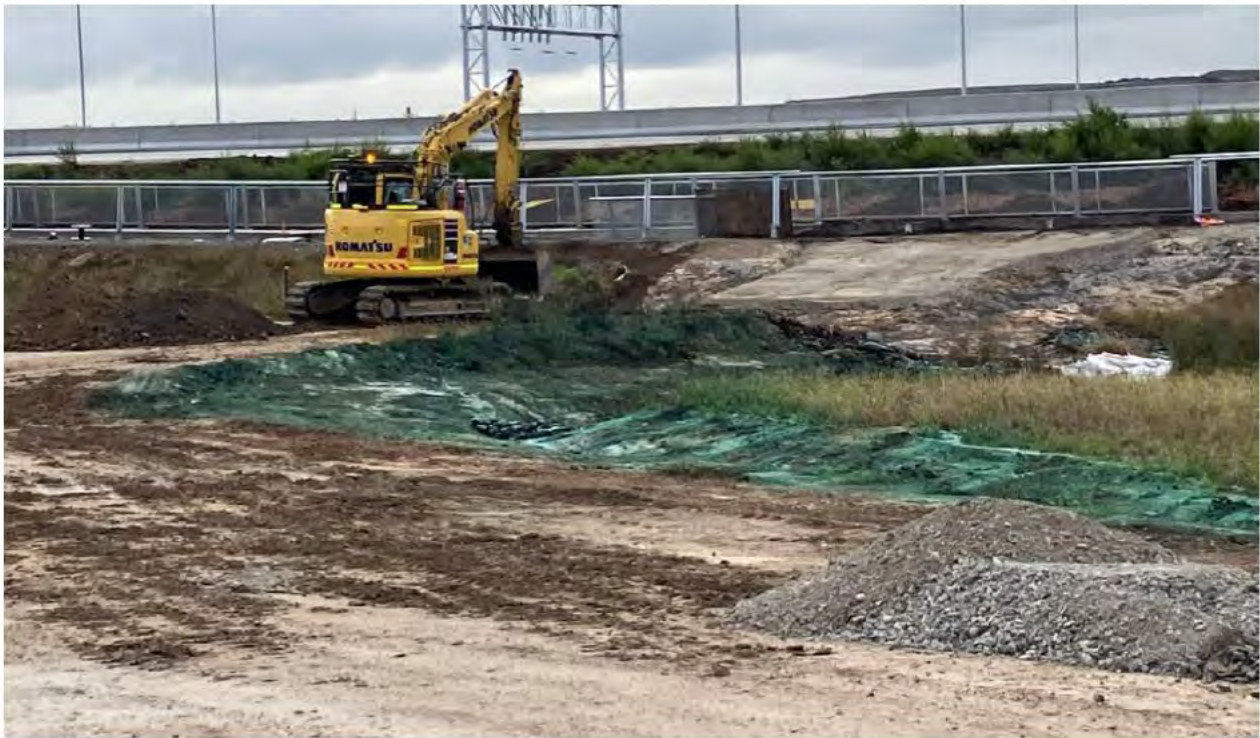
Batter works for seeding. Areas polymer sprayed.
