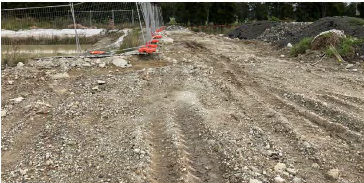
M12C-06_OBS-01 (Ancillary Facility): Water diversion to be improved upon – construction of channels to manage the flow of dirty water required to prepare the site for use at AF12a.
