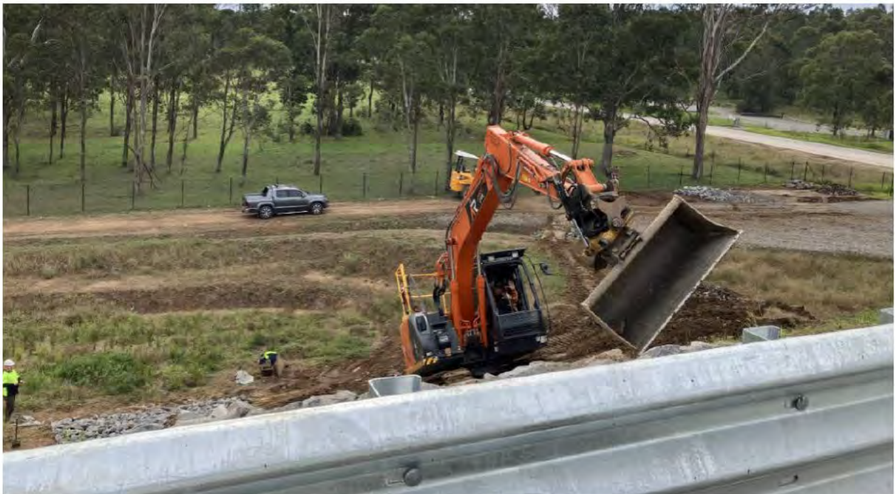
Batter rectification as chutes were missing steel reinforcements
