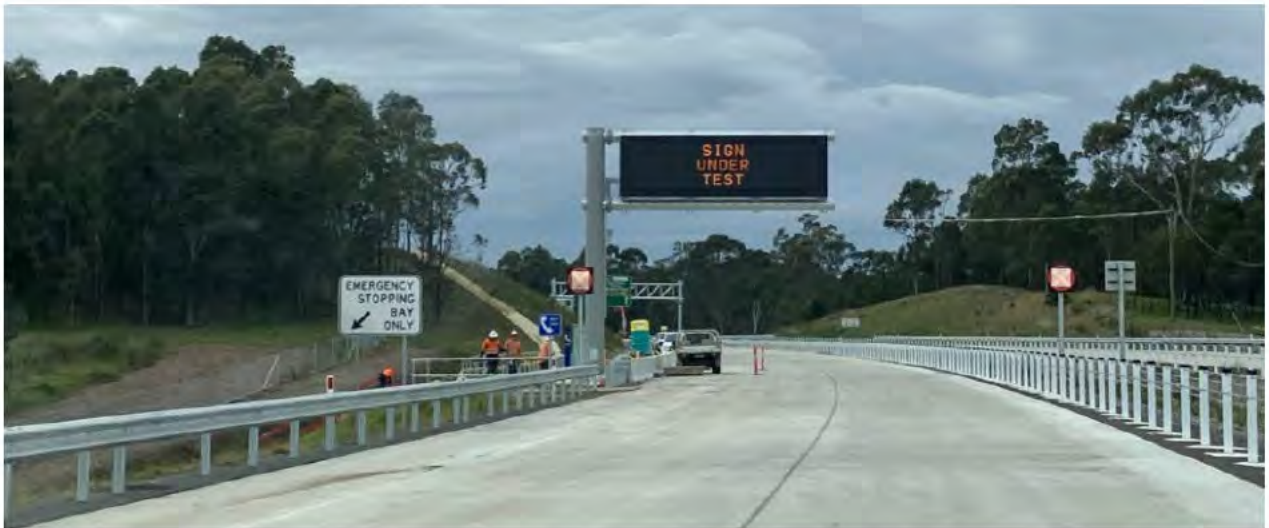
VMS board undergoing testing
