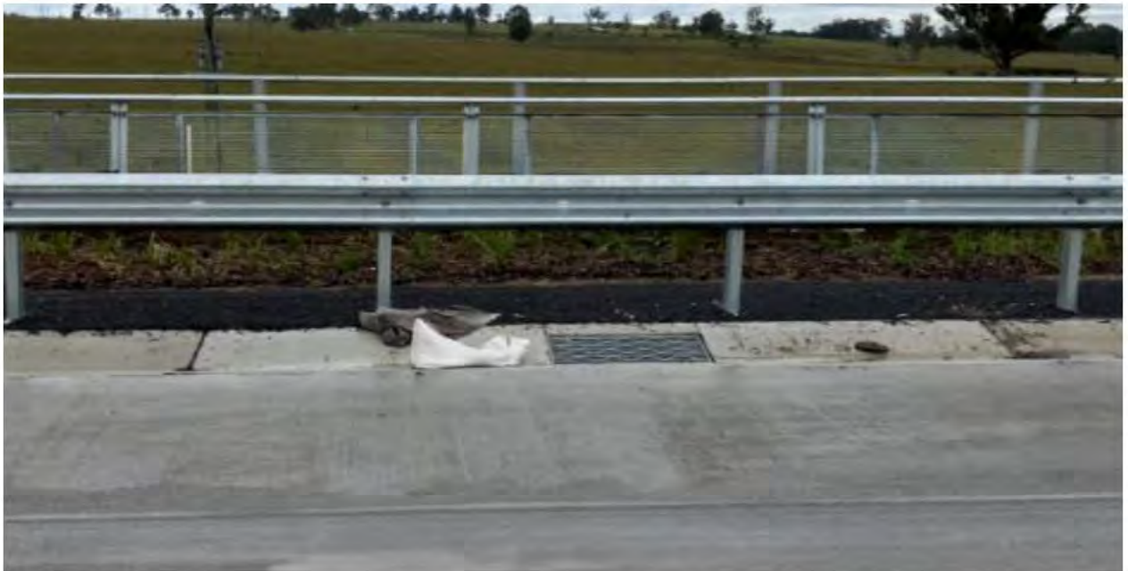
M12W-06_OBS-01: Displacement of sandbags throughout the site requiring removal or reinstatement as required.
