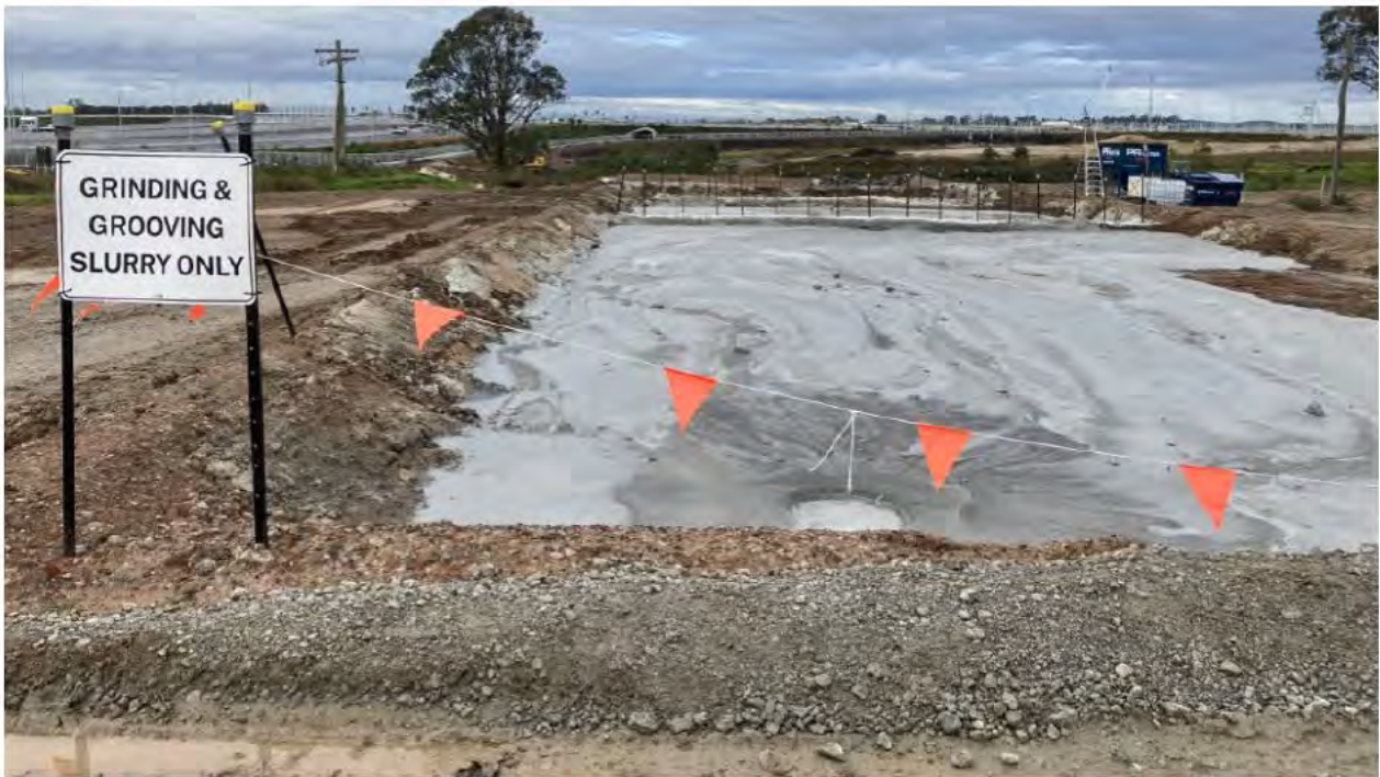
Slurry catchment with signage.
