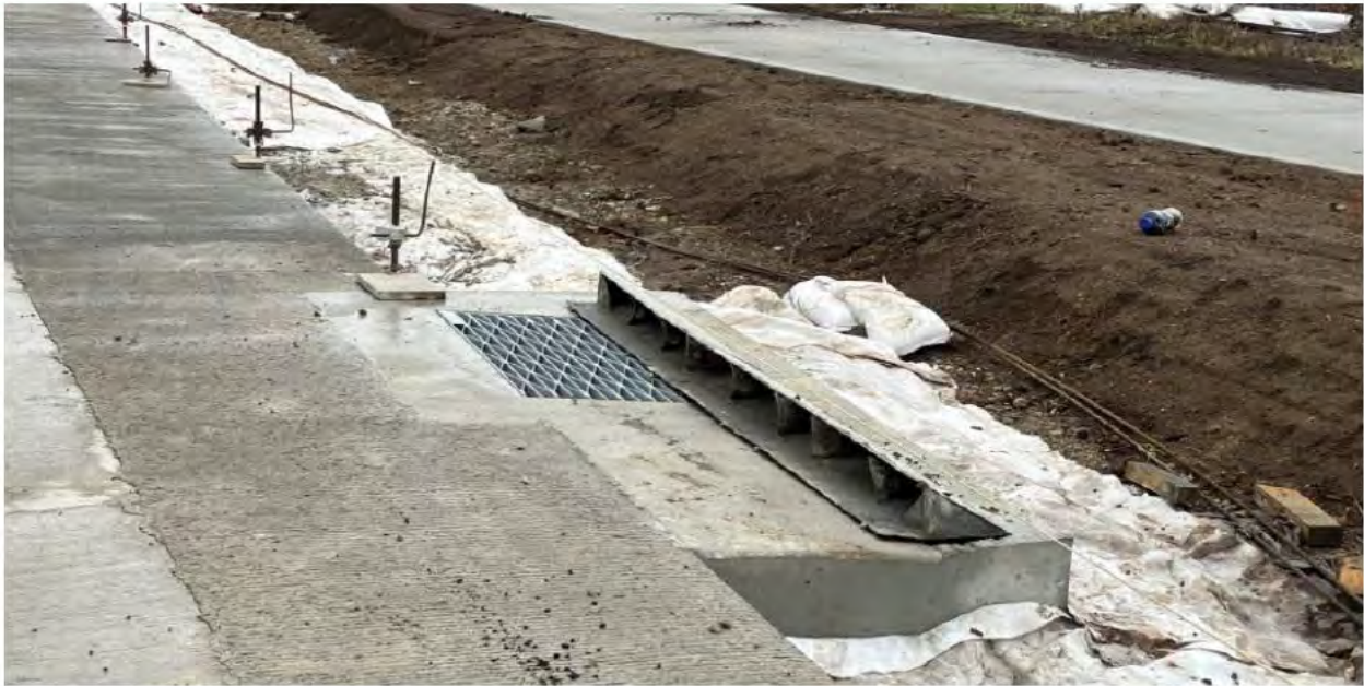
M12W-06_OBS-01: Live drain missing protection; controls required as barrier works were occurring in this area.
