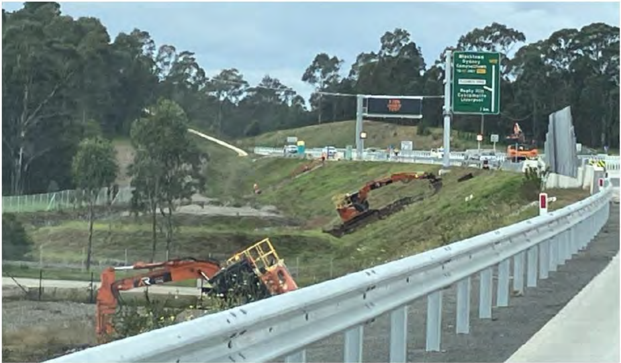
Batter chute rectification works occurring at the time of the audit site inspection
