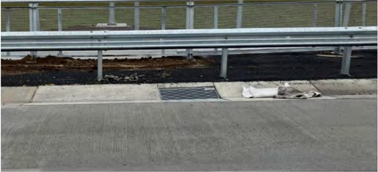
M12W-06_OBS-01: Displacement of sandbags throughout the site requiring removal or reinstatement as required.
