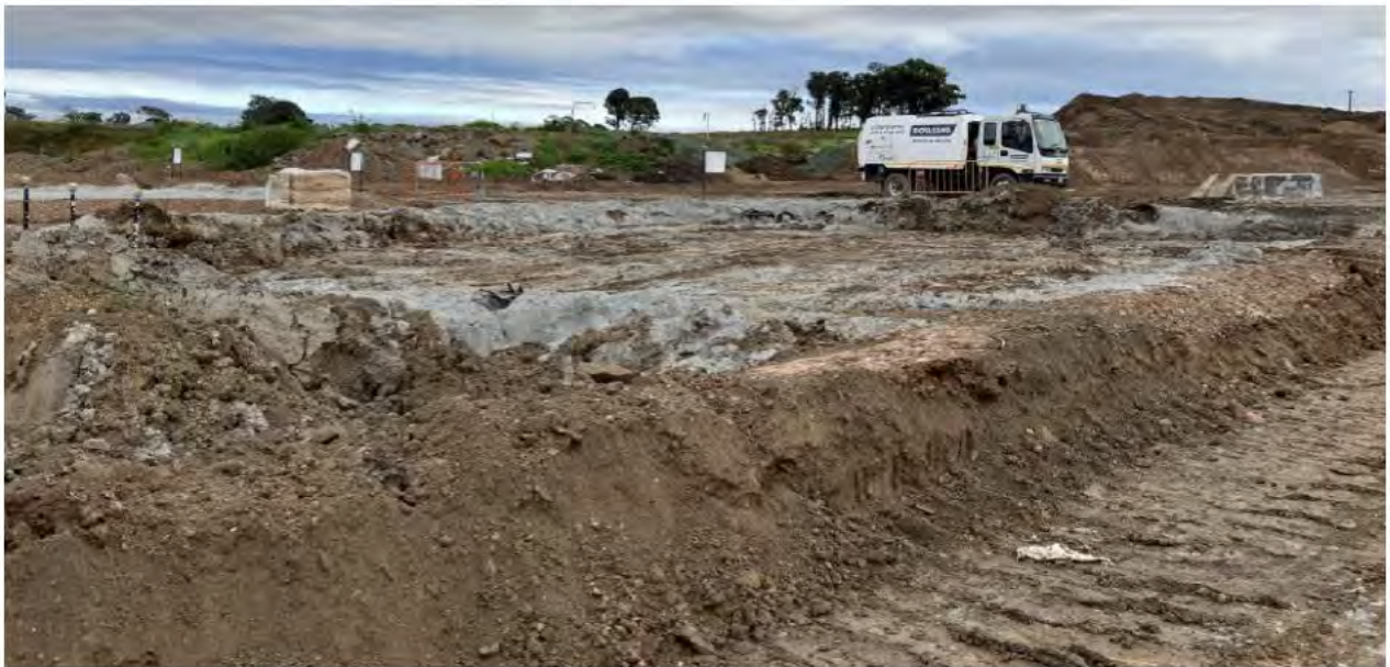
Slurry material drying out for reuse
