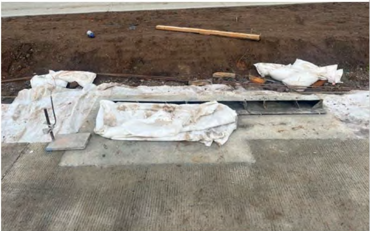
M12W-06_OBS-01 (Close out): Photo provided showing drain covered with geofabric (noted that sandbags unable to be installed due to upcoming use of the slip-form paver).
