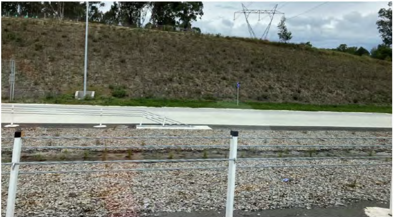
Mulch being removed and will be replaced with a grass lined median strip
