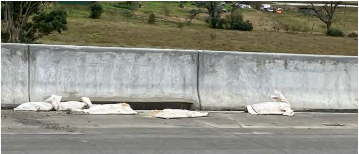
M12W-06_OBS-01: Displacement of sandbags throughout the site requiring removal or reinstatement as required.
