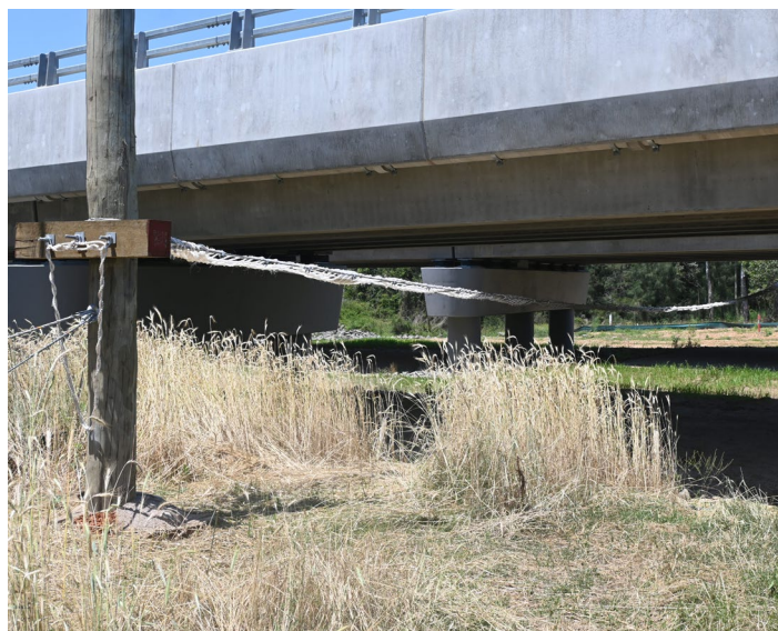
Fauna rope crossing under the new Kemps Creek bridge
