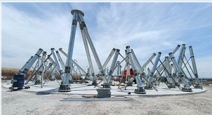
Installing the steel columns
