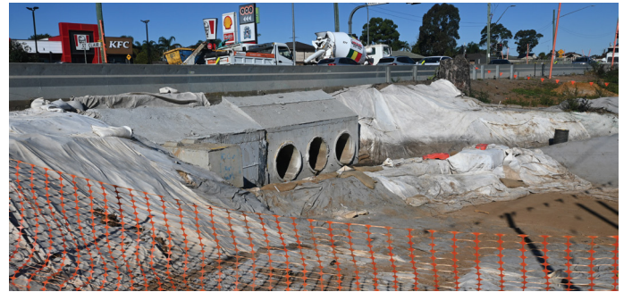
Stormwater connection to GPT
