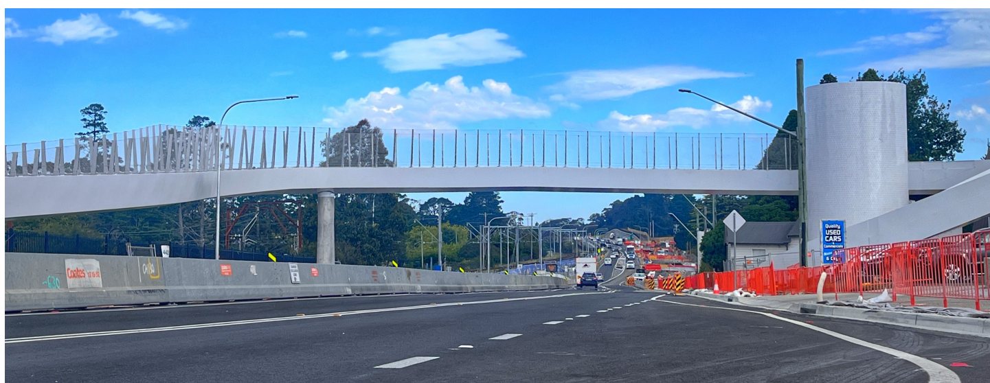
Pedestrian Bridge lifted into place over the Great Western Highway
