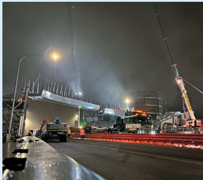
The Pedestrian Bridge being lifted over the highway
