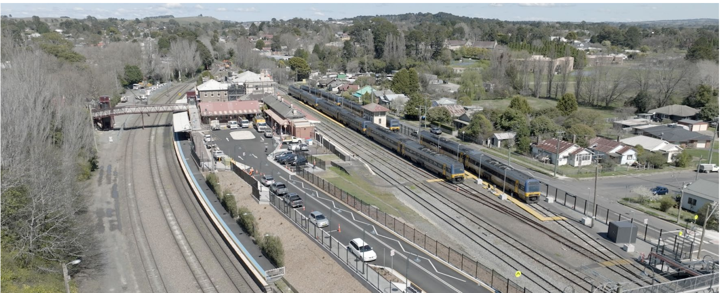
Top photo - The upgraded stabling yard nearing completion. Bottom photo - The temporary stabling yard, opposite Platform 1 at Moss Vale Station, will no longer stable trains once the upgraded stabling yard is completed and handed over.
