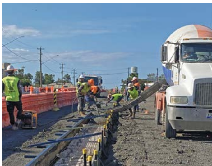
Kerb and guttering work in Bellata
