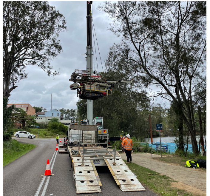
Image: Lifting the drilling rig onto a barge for over-water geotechnical investigations in Wyong River
