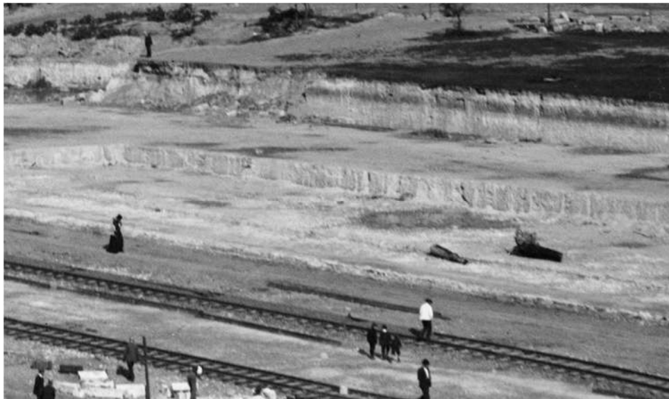
Figure 8-1: Screenshot of a portion of historical photograph taken from Belmore Park area looking south-east, showing stepped excavation for Sydney Terminal building footprint. [picture]. (nla.gov.au)
