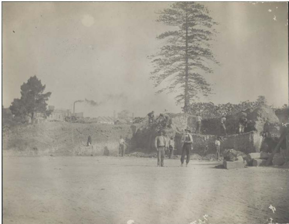
Figure 8-3: Unidentified workers cutting sandstone blocks during the construction of Central railway station, Sydney, 1903? [picture]. (nla.gov.au)
