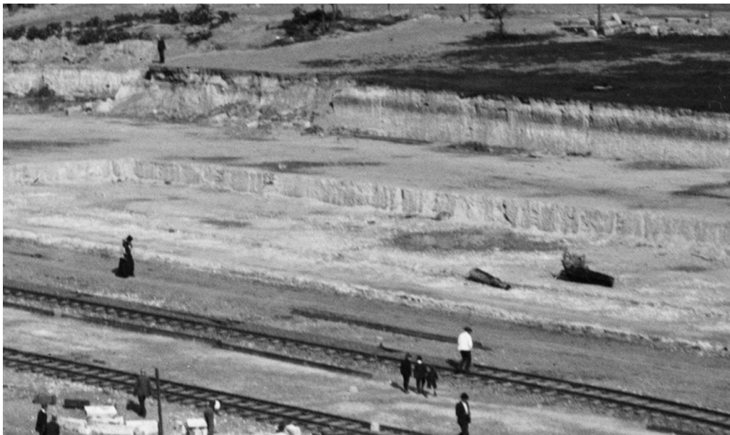
Figure 5-17: Screenshot of a portion of historical photograph taken from Belmore Park area looking south-east, showing stepped excavation for Sydney Terminal building footprint. [picture]. (nla.gov.au)
