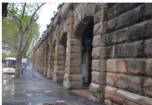
Figure 4-8 Depth of wall constructed on Pitt Street indicating the depth of excavation undertaken to build the ramp up to the Western Forecourt.
