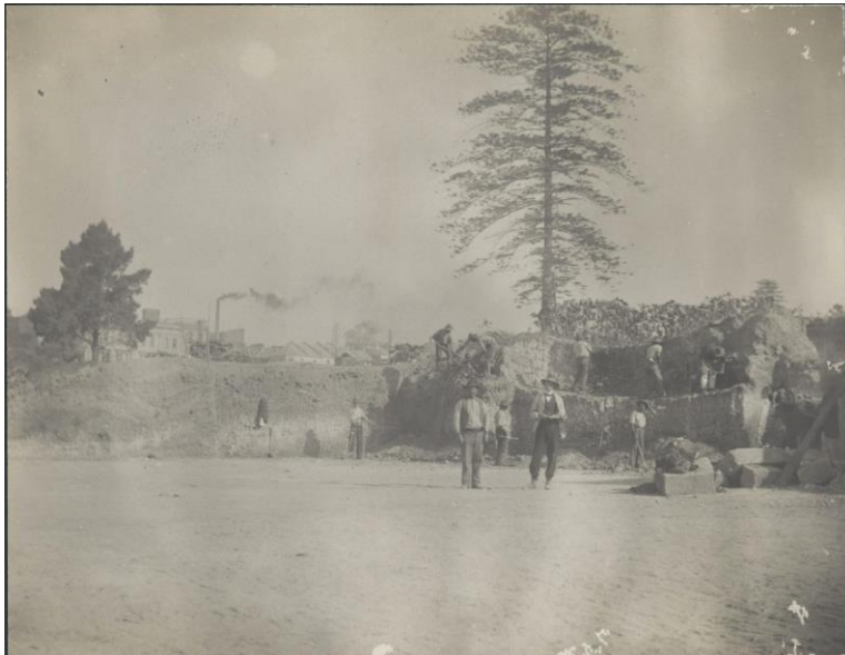
Figure 5-19: Unidentified workers cutting sandstone blocks during the construction of Central railway station, Sydney, 1903? 63
