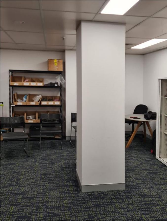
62 Encased columns within offices Source: TKD Architects, May 2022
