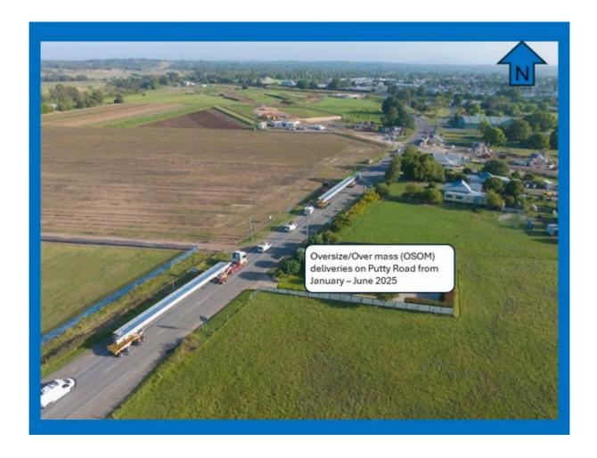
Oversize/Overmass (OSOM) vehicles will be making regular deliveries of concrete headstocks and girders along the project alignment. Example above is a delivery of girders (32m in length) using Putty Road.
