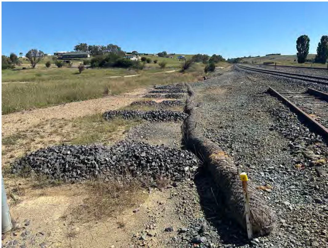
Photo 13: Rock armoury in drainage channel between southern and middle culverts appears to be in good condition.
