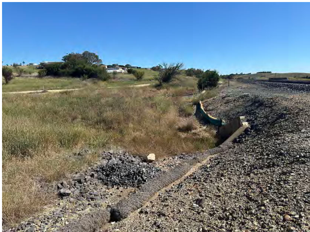
Photo 14: Sediment controls at the middle culvert upgradient of the railway line in good condition.
