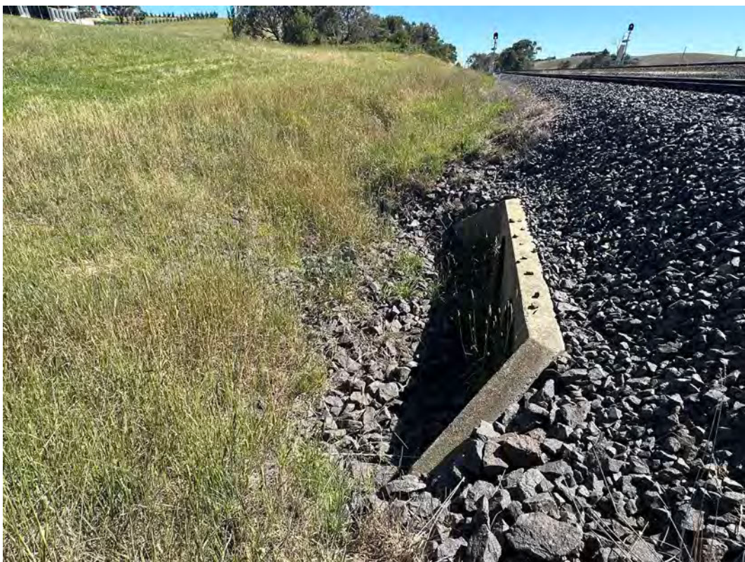
Photo 18: Upgradient of northernmost culvert with no surface water. No sediment build up was noted on rock armoury.
