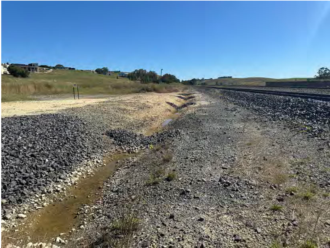
Photo 17: Rock armoury in drainage channel between middle and northern culverts appears to be in good condition.
