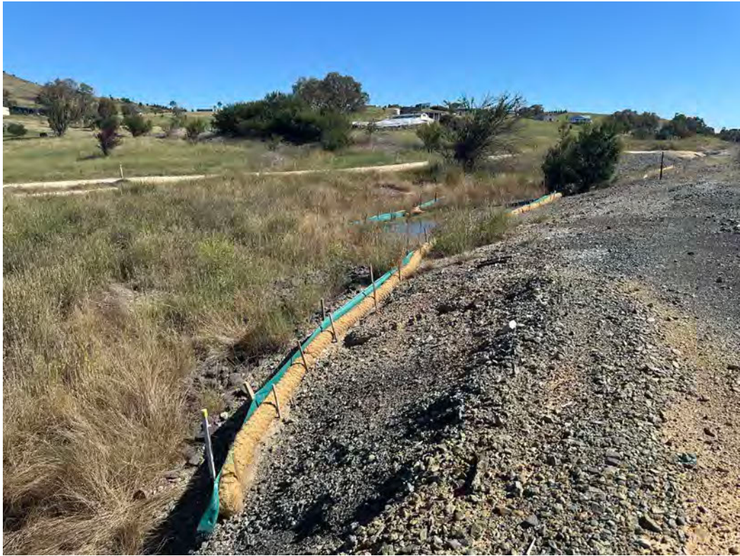
Photo 15: Sediment controls north of middle culvert, upgradient of railway line in good condition. Minor inadequate ground cover observed during the previous inspections remained in a stable condition.
