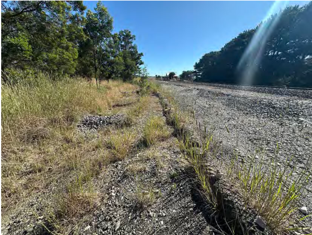
Photo 11: Rock armoury in drainage channel between southern and middle culverts replenished and less sediment and vegetation build up observed.
