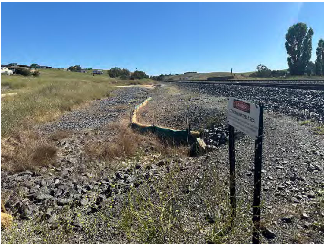
Photo 16: Sediment controls in drainage channel between middle and northern culverts appears to be in good condition.
