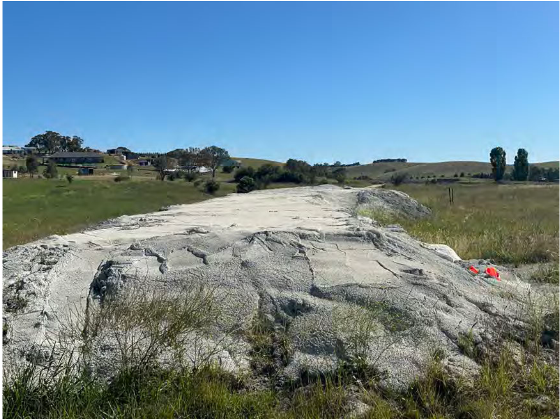
Photo 19: The concrete-capped stockpile is generally in good condition with no new erosion observed.
