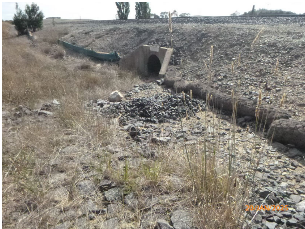
Photo 12: Sediment controls at the middle culvert upgradient of the railway line in good condition.
