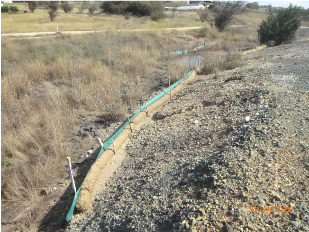
Photo 13: Sediment controls north of middle culvert, upgradient of railway line in good condition. Sediment buildup in front of coir logs increased since last inspection.
