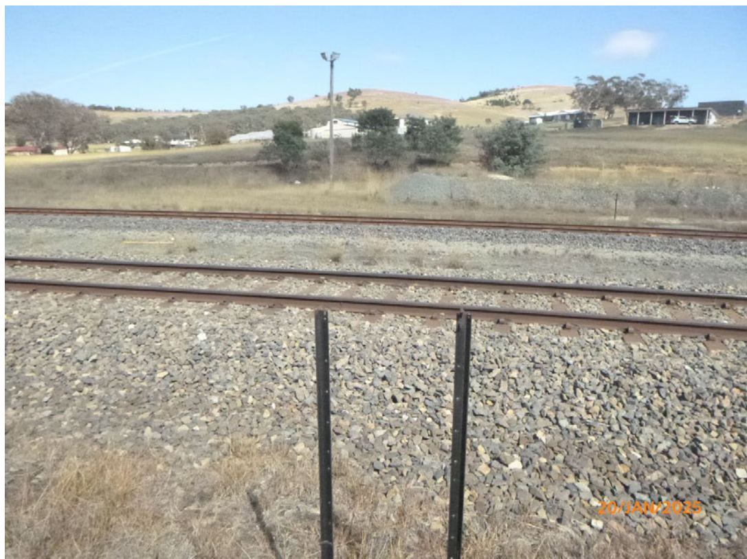
Photo 20: One exclusion zone sign missing. Signage approximately 100 north on eastern side of rail.
