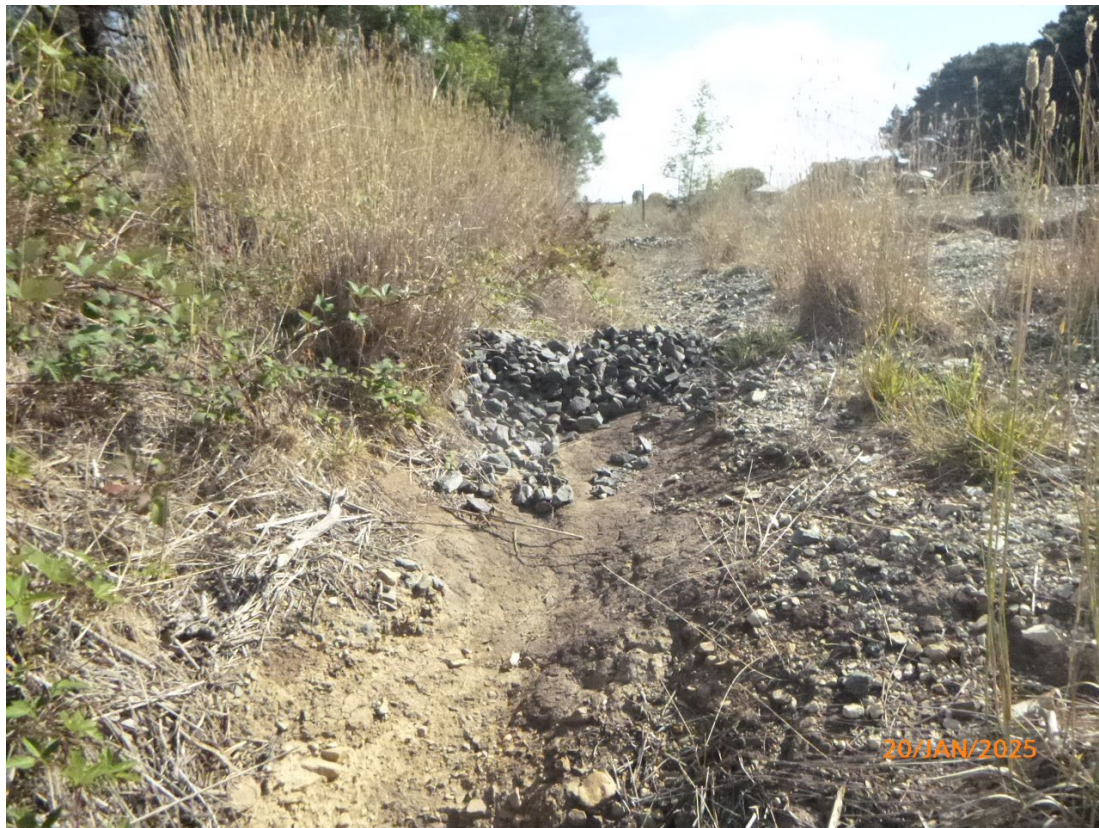
Photo 9: Rock armoury in drainage channel between southern and middle culverts. Sediment and vegetation buildup minimal within drainage line.
