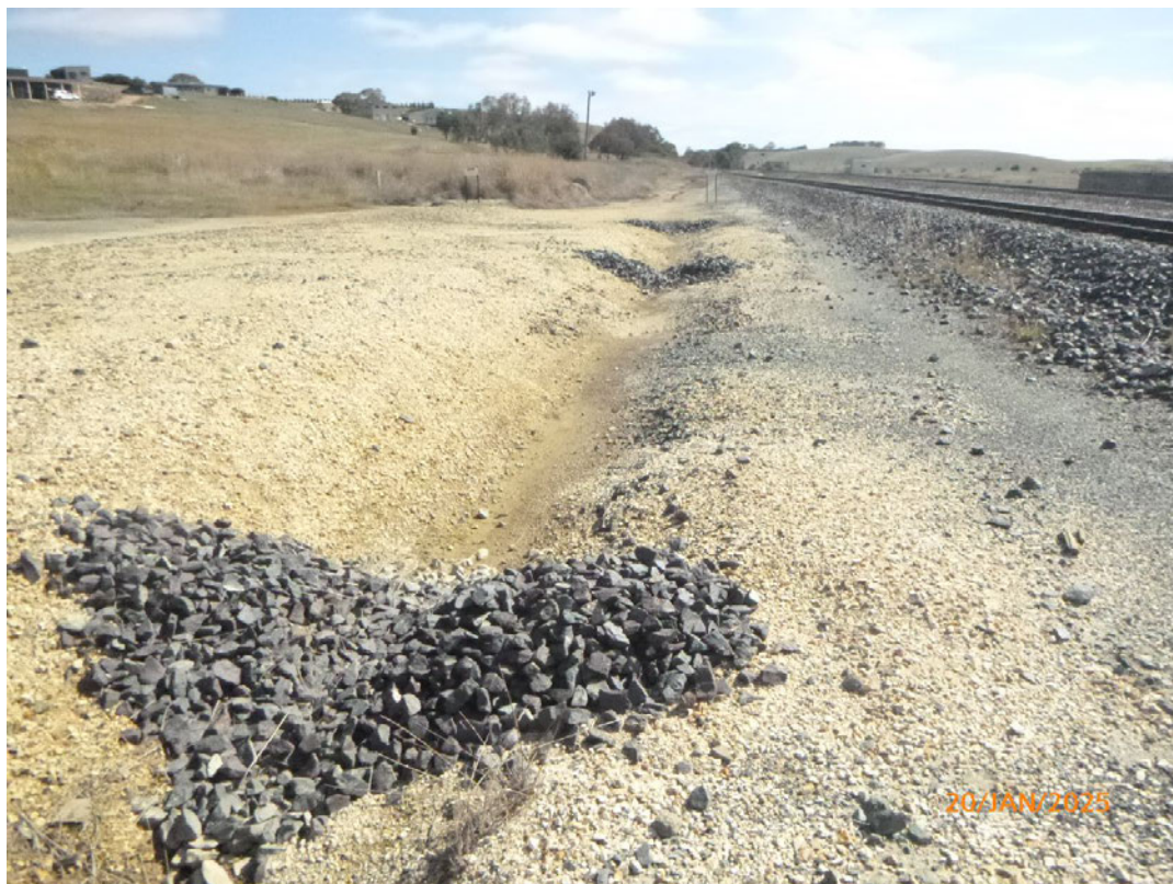
Photo 15: Rock armoury in drainage channel between middle and northern culverts appears to be in good condition.
