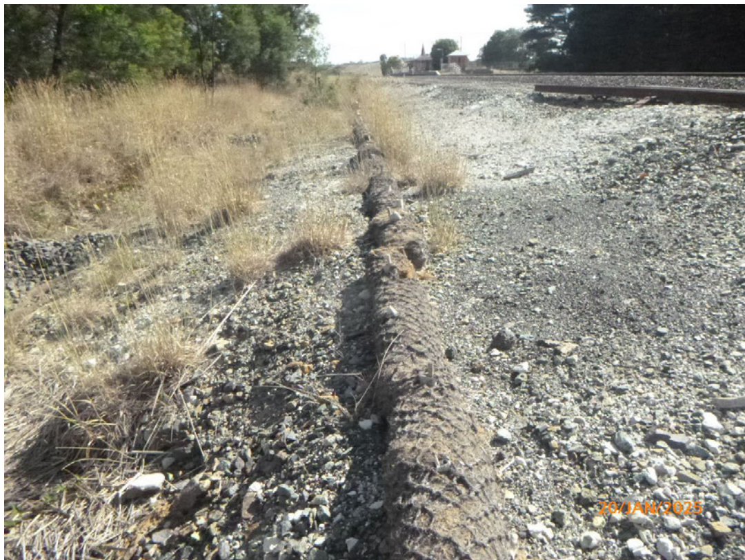
Photo 8: Sediment controls at southernmost culvert upgradient of the railway line.
