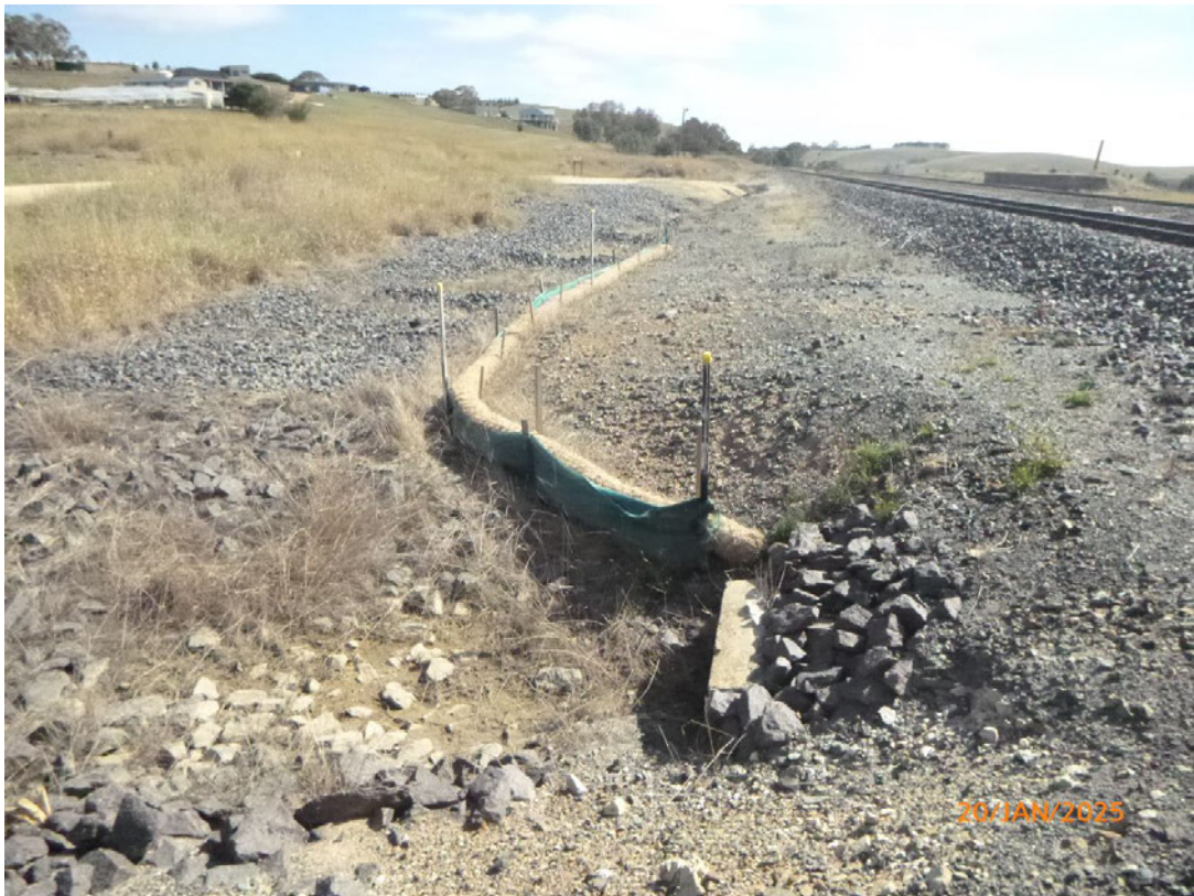
Photo 14: Sediment controls in drainage channel between middle and northern culverts appears to be in good condition.
