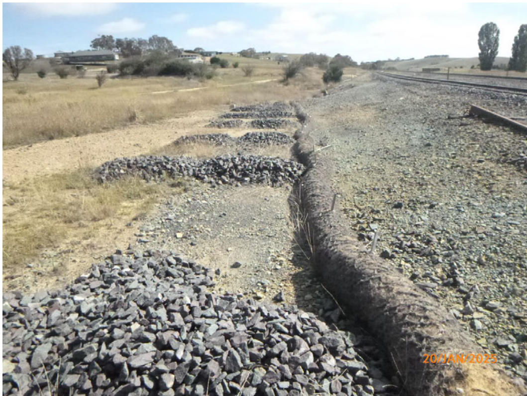
Photo 11: Rock armoury in drainage channel between southern and middle culverts appears to be in good condition.
