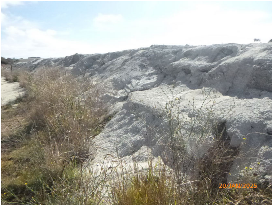
Photo 17: The concrete-capped stockpile is generally in good condition with no new exposure locations observed.
