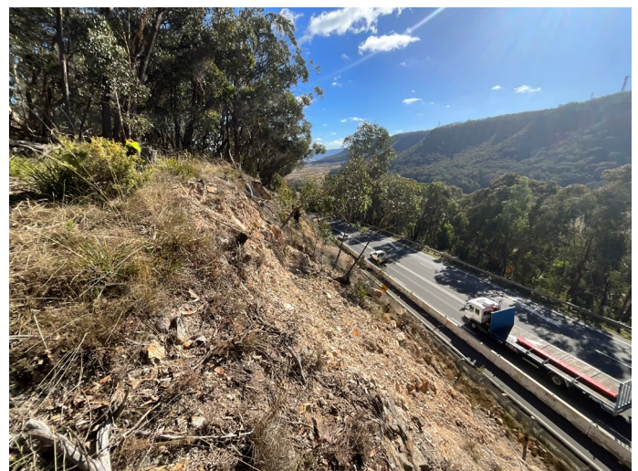
Upslope failure on the Great Western Highway at Victoria Pass
