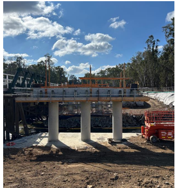
Piling for the new Warroo Bridge is complete and the bridge columns and headstocks are ready for the Super T girders to be craned into place in July
