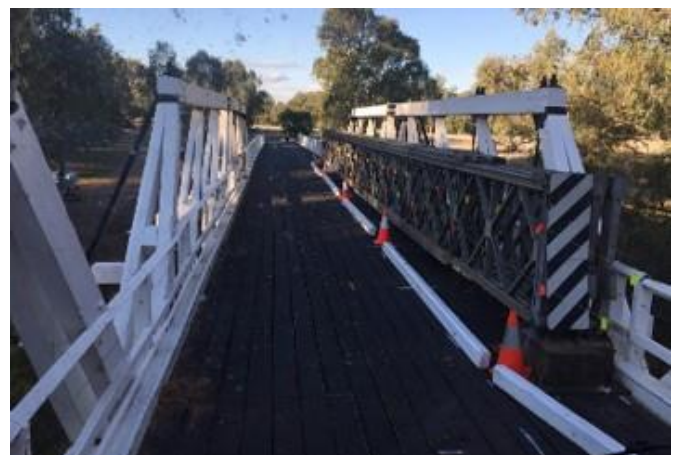
A Bailey bridge has been used at Paytens Bridge at least three times since 2000, most recently in 2017 (pictured) following overloading issues which required the bridge to be closed for a month.
